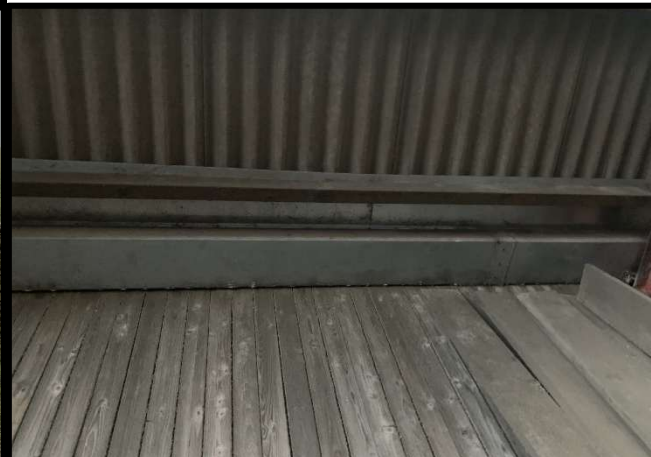
Photograph 4. Internal agricultural barn.
