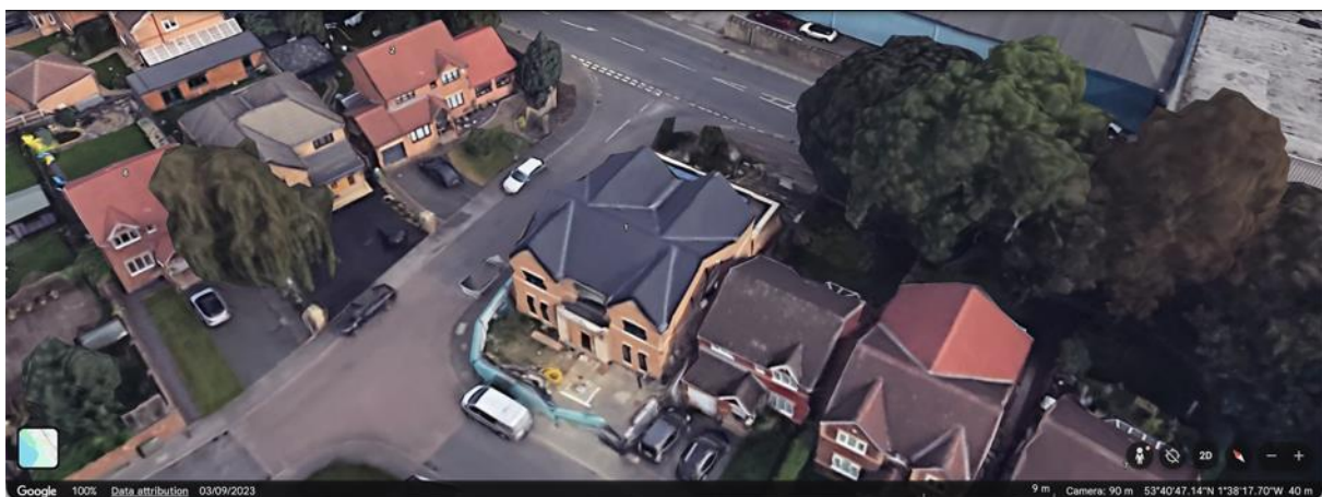
Image 1 – Examples of approved residential front, side and rear extensions on Old Mill View 2020/91133 - Erection of extensions, external alterations and conversion of integral garage to living accommodation; &
