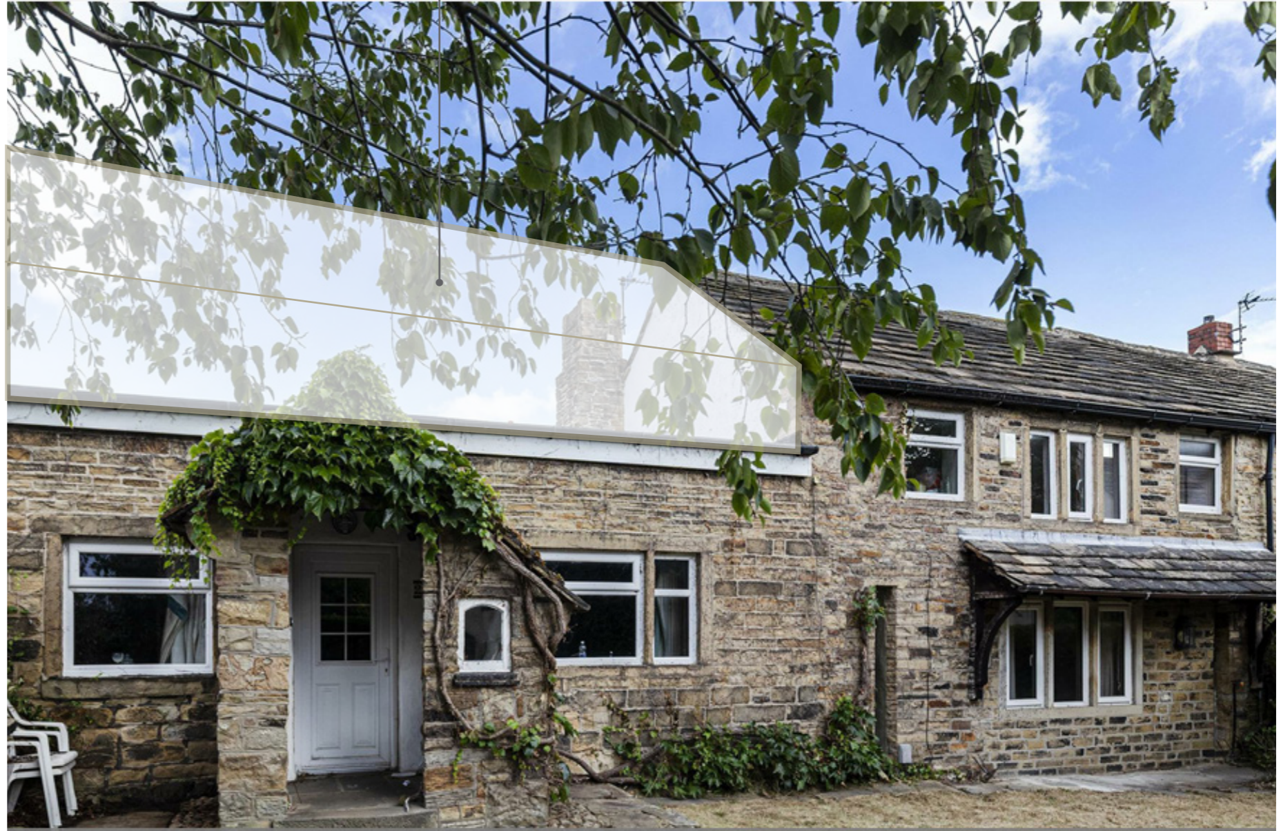
View looking North into the site from Rowley Hill indicating the reinstatement of the former first floor and pitched roof.
