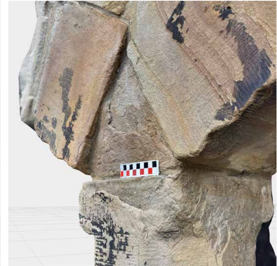
Photogrammetry of the Voussoirs associated with the coach house arch, showing the cut of stone and attention to detail through splays and triangular capital head.
