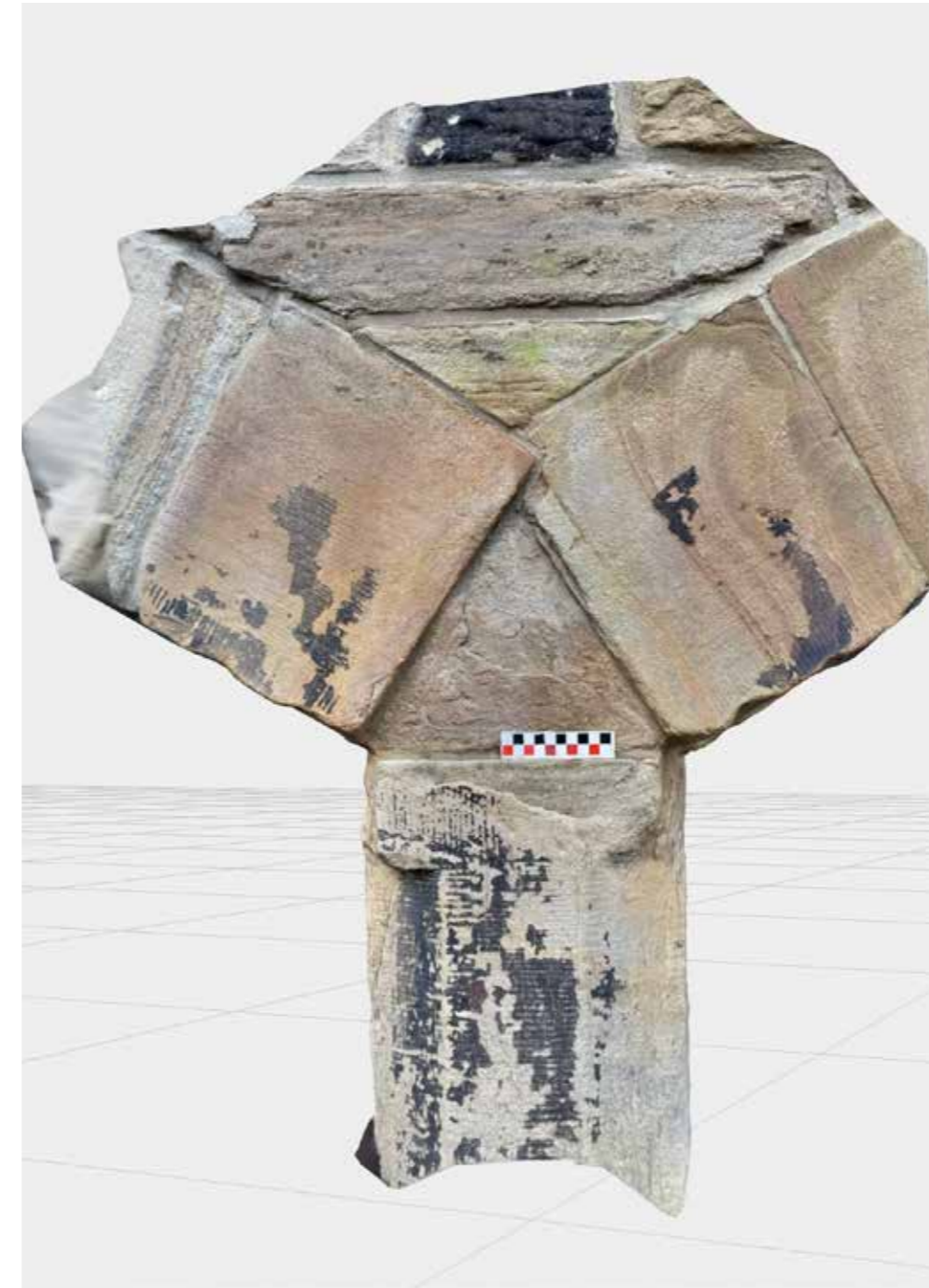
Photogrammetry of the Voussoirs associated with the coach house arch, showing the cut of stone and attention to detail through splays and triangular capital head.
