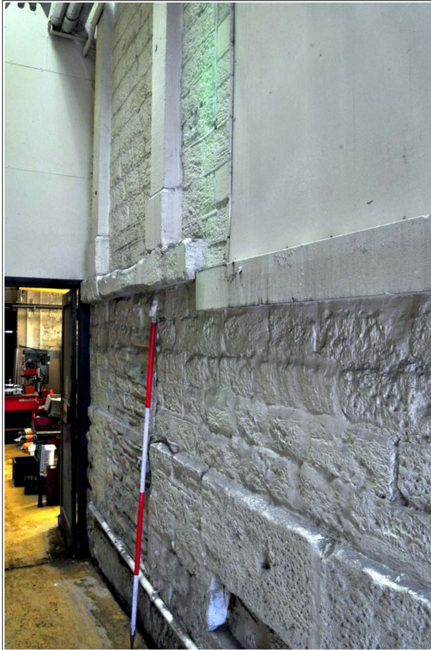
05: Foot of former doorway, north elevation, looking east
