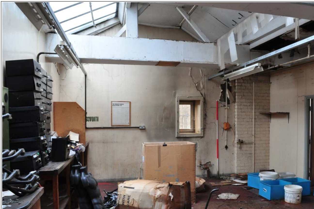
16: Second floor, looking south
