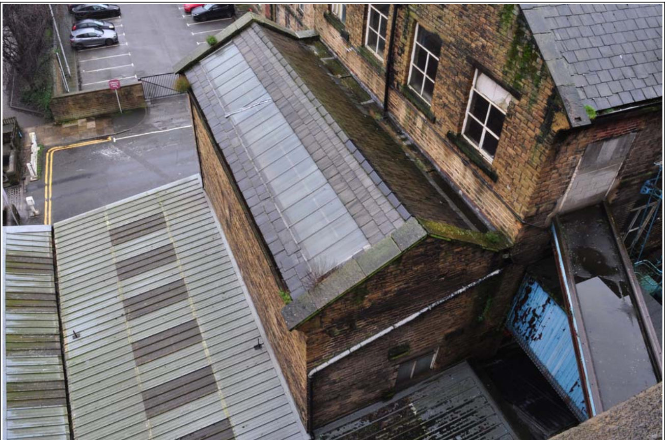
11: View of roof, looking south-west
