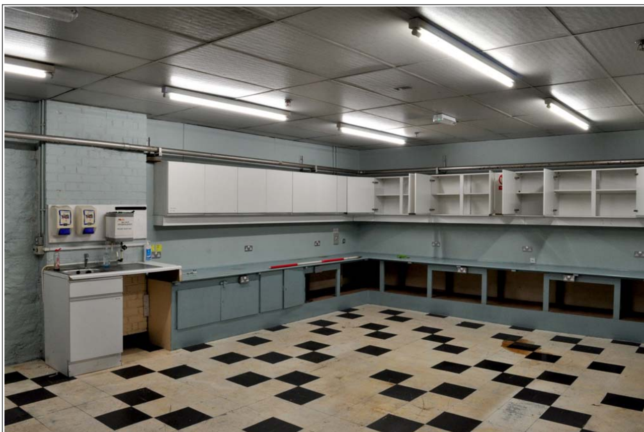
13: Ground floor, looking north-east
