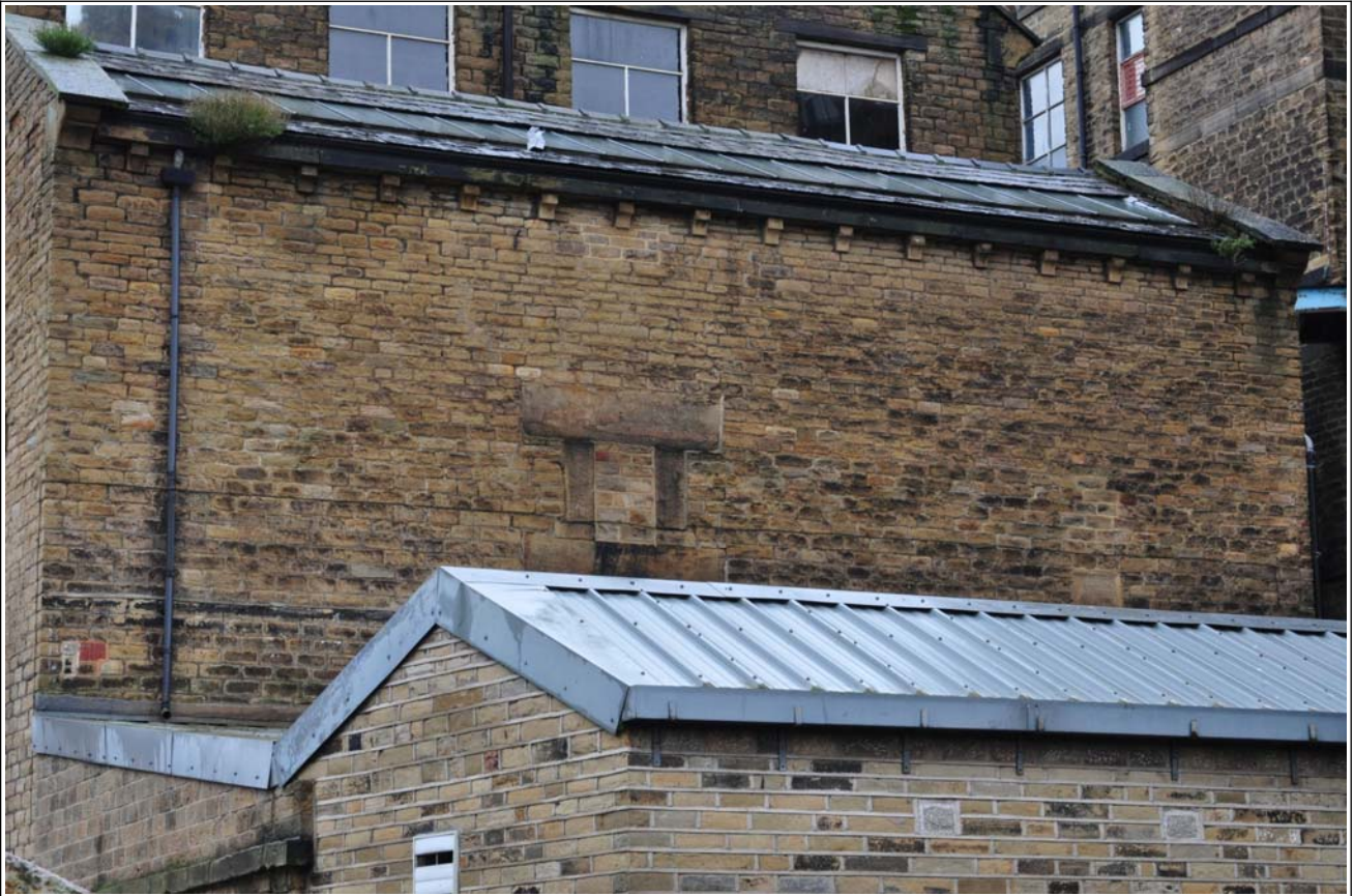
10: East elevation above former boiler house, looking north-west
