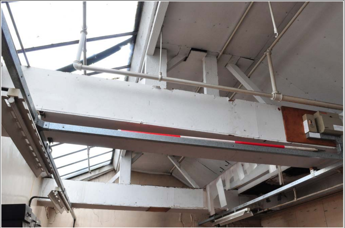
18: Roof structure, looking south
