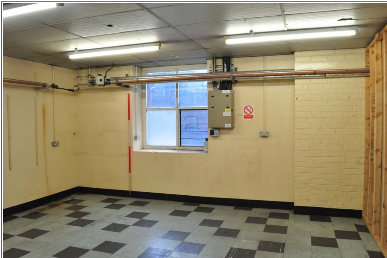
12: Ground floor, looking south-east
