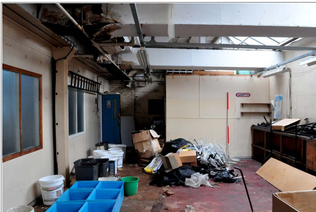
17: Second floor, looking north
