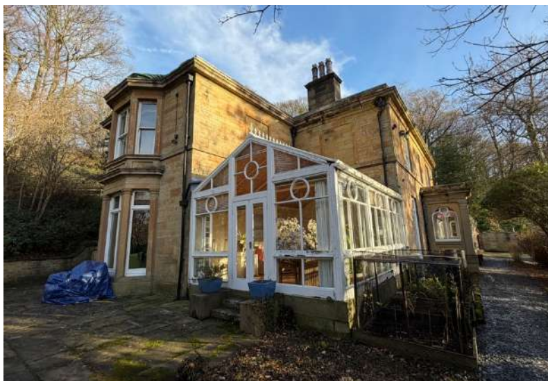
Figure 4.5: West Elevation, Parkton Grove (December 2025)
