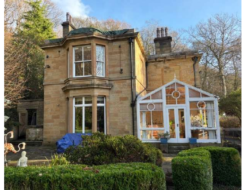
Figure 4.4: West Elevation, Parkton Grove (December 2025)
