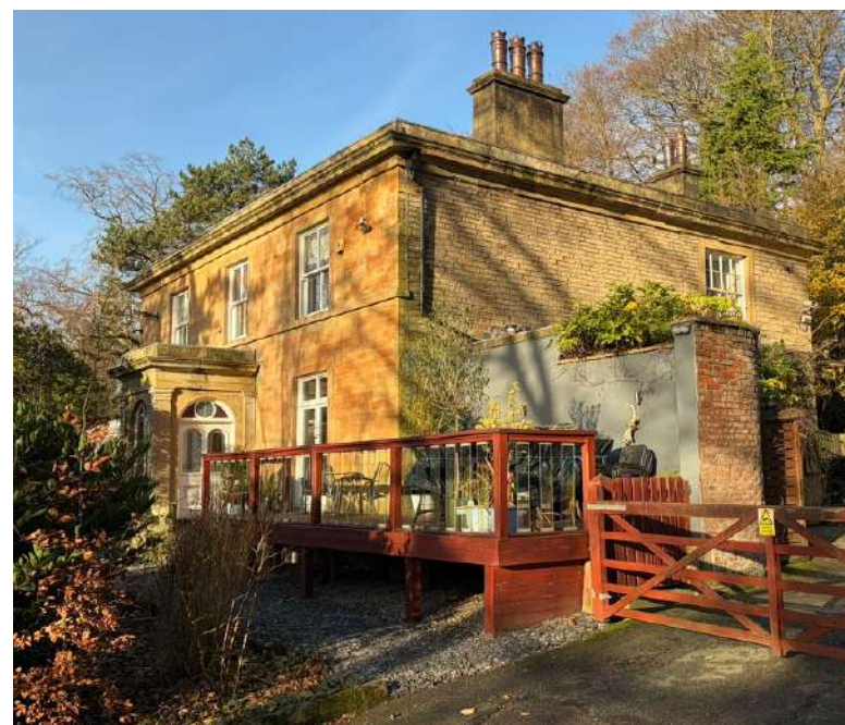
Figure 4.2: South and East Elevations, Parkton Grove (December 2025)
