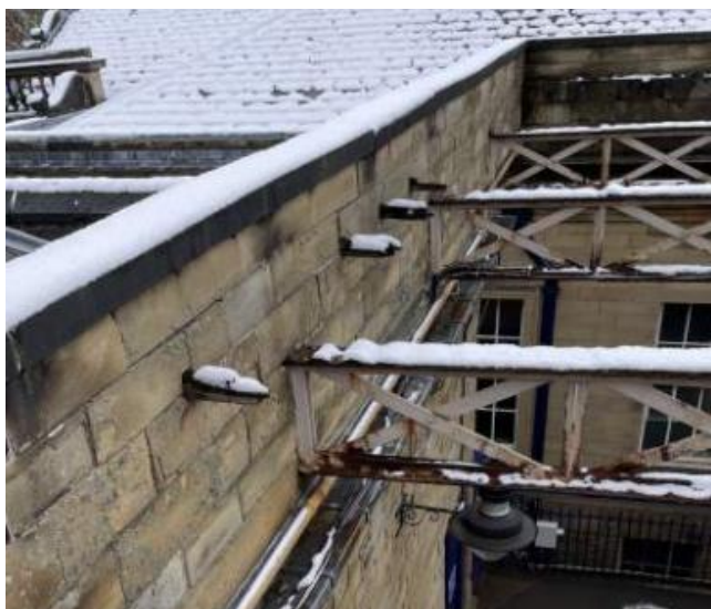
Insert 4-19 – Photos showing the surviving lateral trusses and evidence of the cut off previous roof covering, where the drivers’ welfare building had been connected laterally to Roof A.
