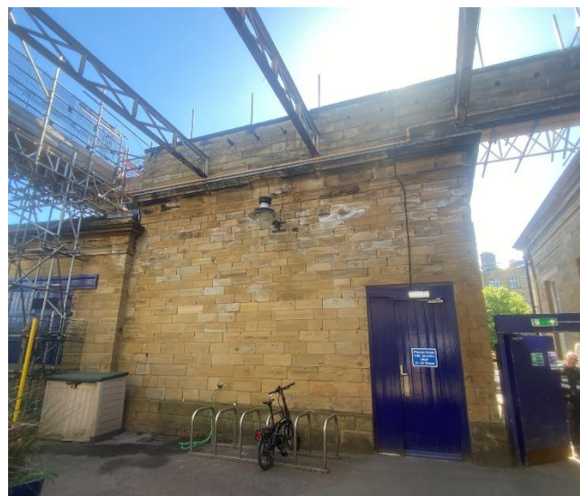
Insert 4-19 – Photos showing the surviving lateral trusses and evidence of the cut off previous roof covering, where the drivers’ welfare building had been connected laterally to Roof A.
