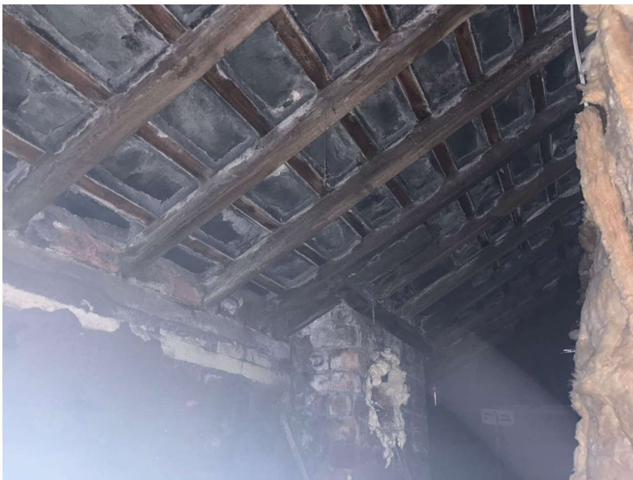
Figure 5 - Internal view of unconverted loft area B1
