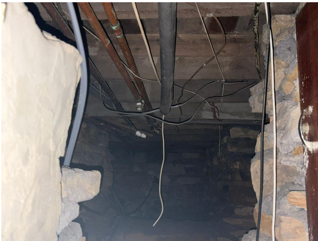
Figure 4 – Internal view of unconverted loft area B1
