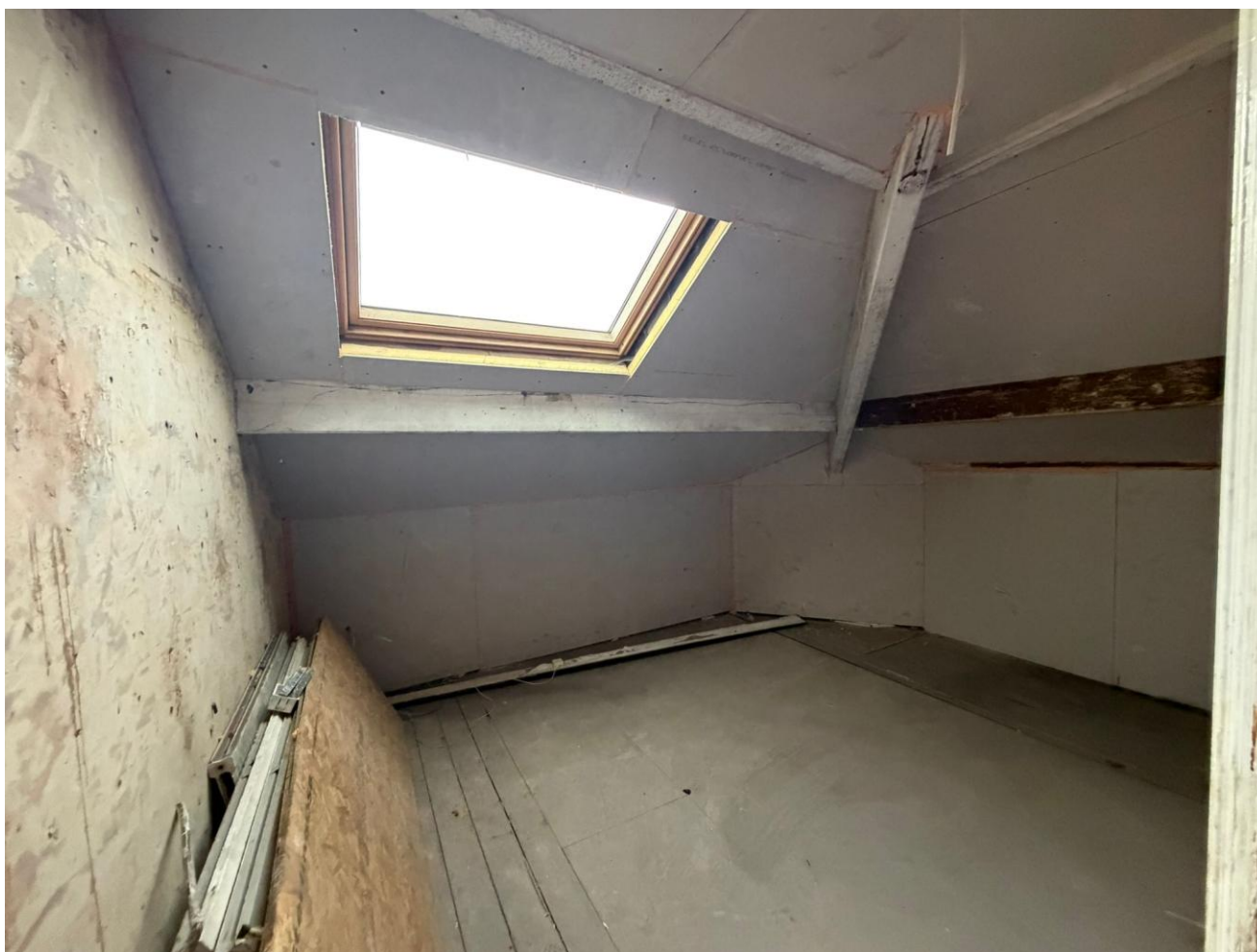
Figure 6 – Internal view of converted loft space
