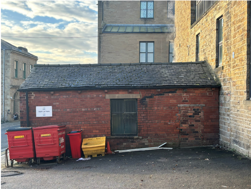
Figure 12 - The North Elevation - Note the garages abutment to the listed building
