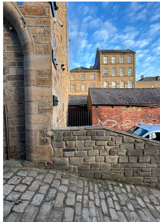
Figure 15-The connection between the wall and the listed building
