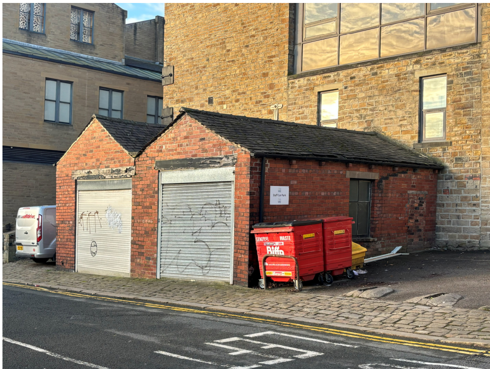
Figure 11 The existing Garages looking south
