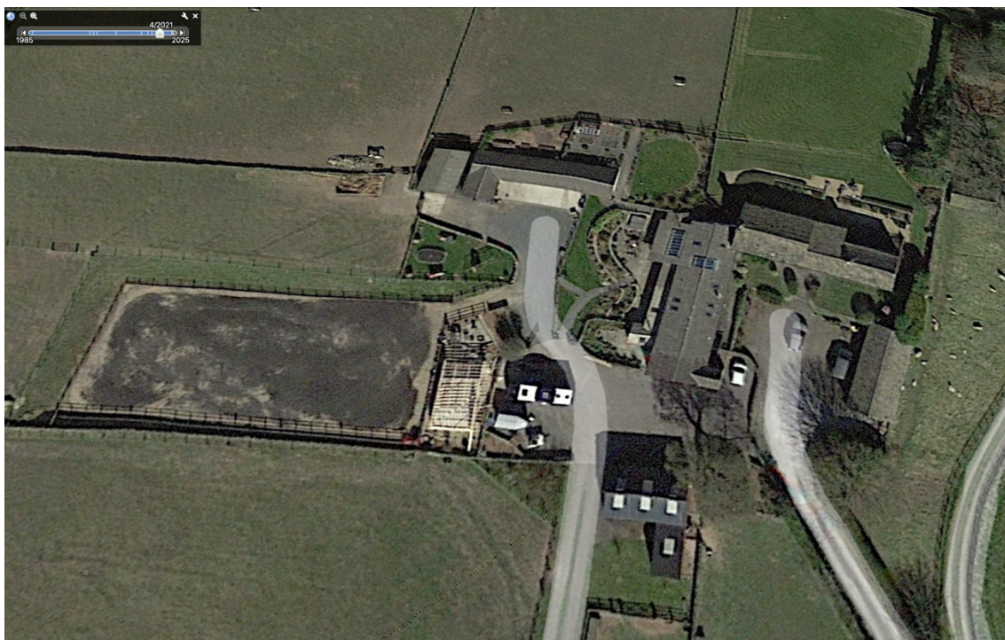
Google Earth Pro screenshot - construction of the building taking place in April 2021 – over 4 years ago
