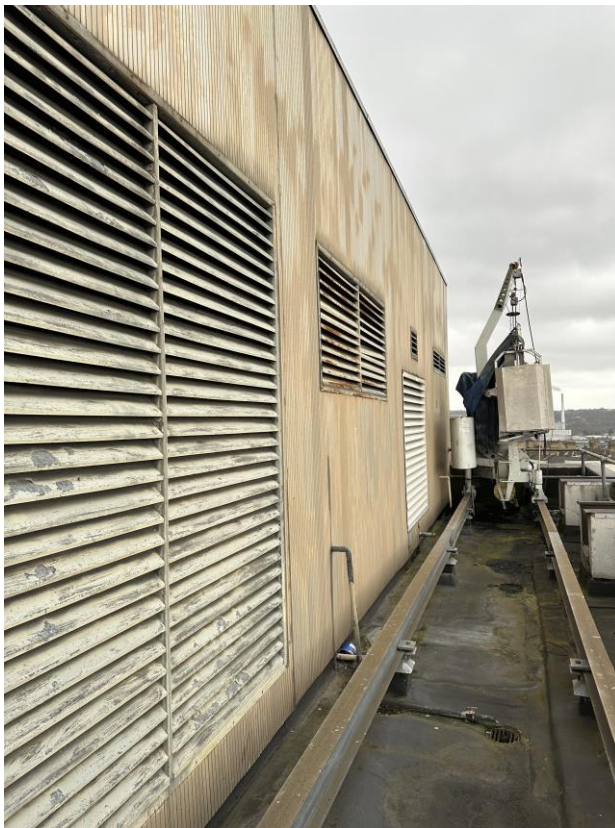
Photograph 3 – Existing cladding on sixth floor
