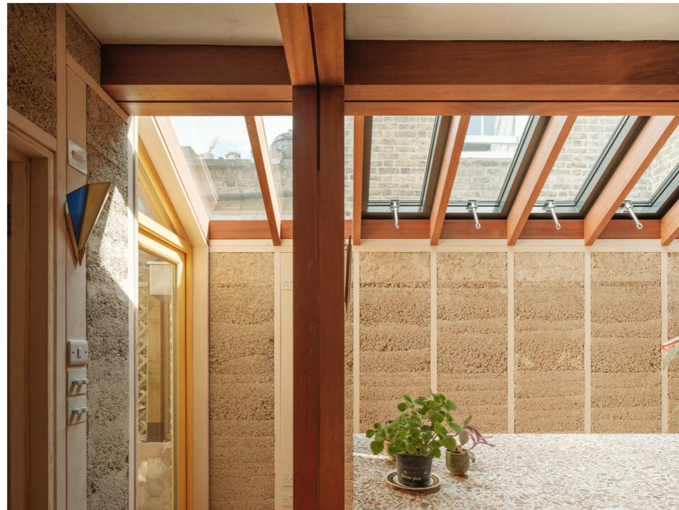
image showing an example of timber frame and hempcrete construction method which will be used to construct the extension
