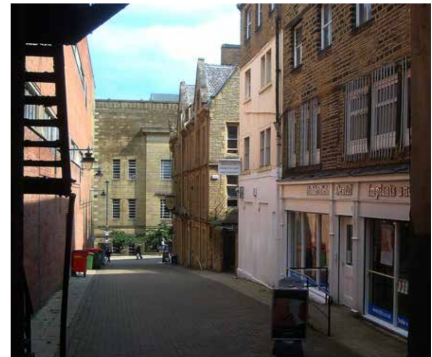
4.3.8 - View of west elevation from Albert Yard
