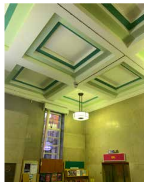
4.5.3 - Ceiling to Entrance Lobby / Reception (Rm.52)
