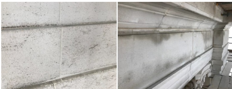
Plate 9: Examples of a completed system with the CP anodes chased and over mortared, albeit in a Portland stone façade. 37
