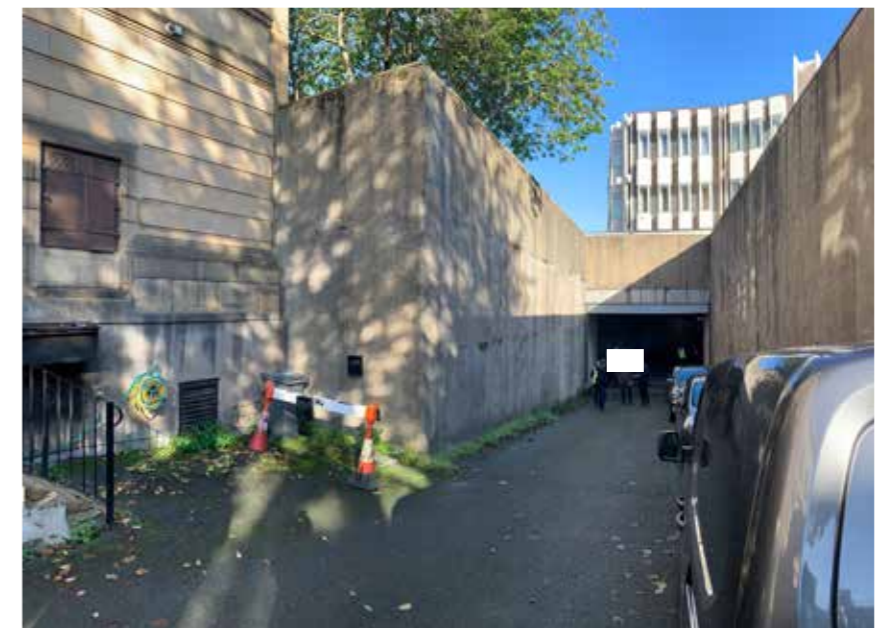
4.4.7 - Tunnel access below east elevation
