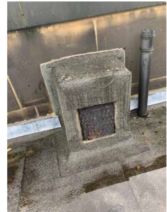
4.4.18 - Service access at roof
