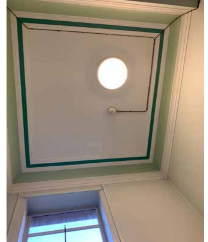
4.6.4 - Ceiling to First Floor Stair Lobby (Rm.71)
