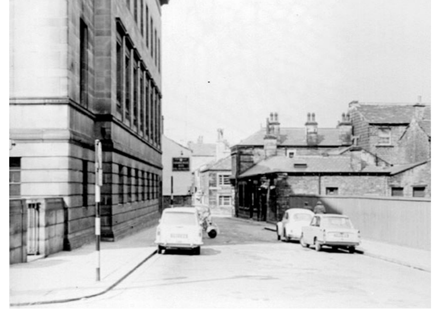
4.2.3.9 - East elevation looking onto Bull & Mouth Lane (now lost)
