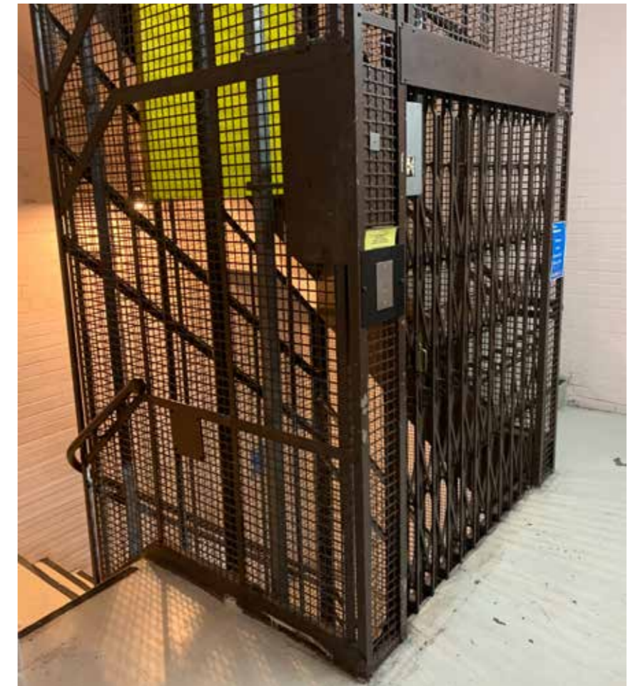
4.5.32 - Stair and Lift (Rm.40 & 41)
