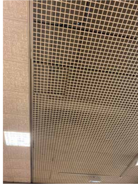
4.7.17 - Ceiling to Gallery 2 (Rm. 86)
