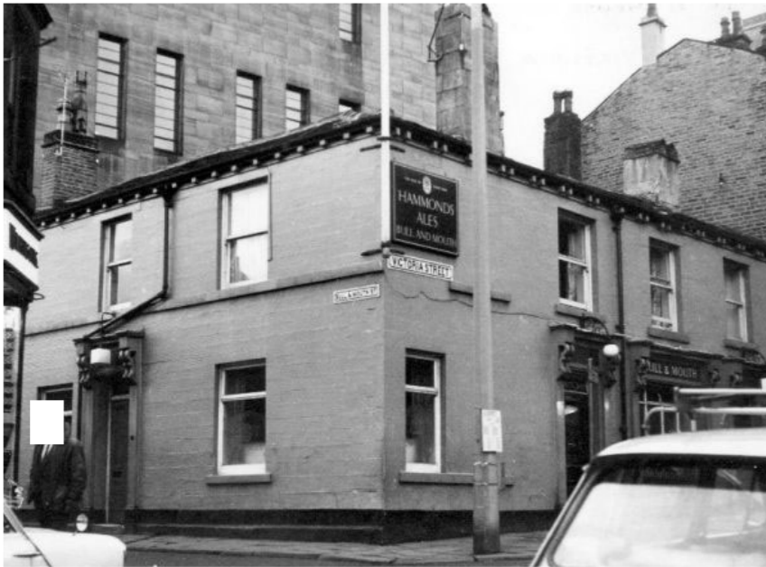
4.2.3.10 - North elevation looking onto Bull and Mouth public house (now demolished), c. early 1960s
