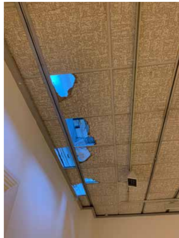
4.7.21 - Ceiling to Gallery 3 (Rm. 85)
