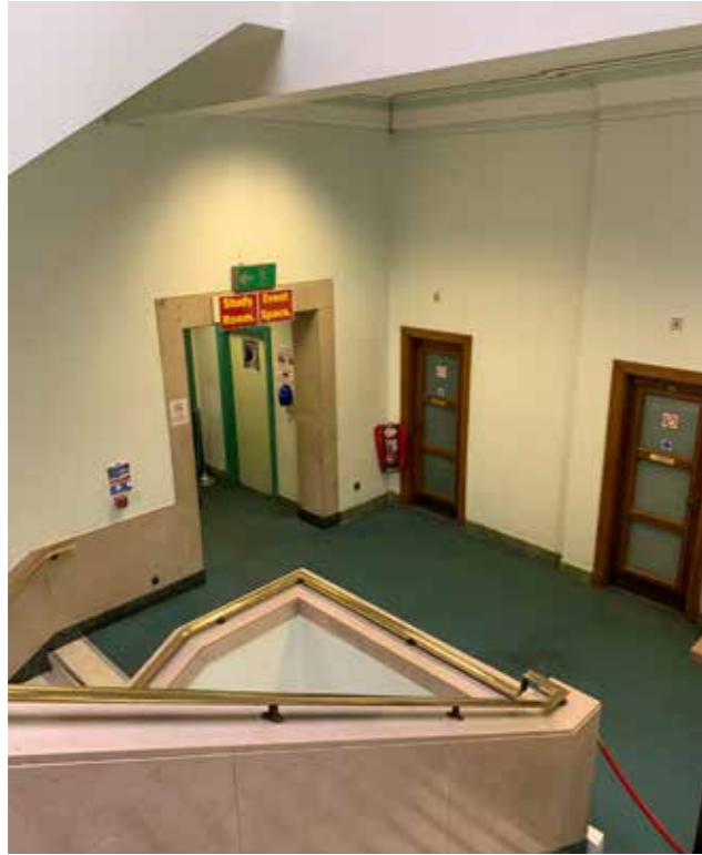
4.6.1 - First Floor Stair Lobby (Rm.71)
