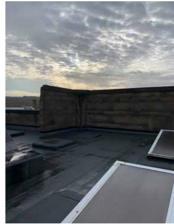
4.4.14 - Modern lanterns to roof
