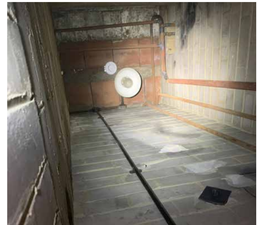
4.7.7 - Plant Space (Rm.89)
