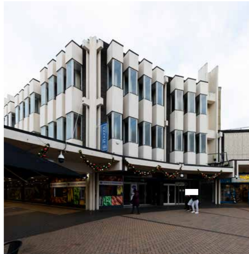
4.3.5 - Piazza Shopping Centre facing building's north aspect
