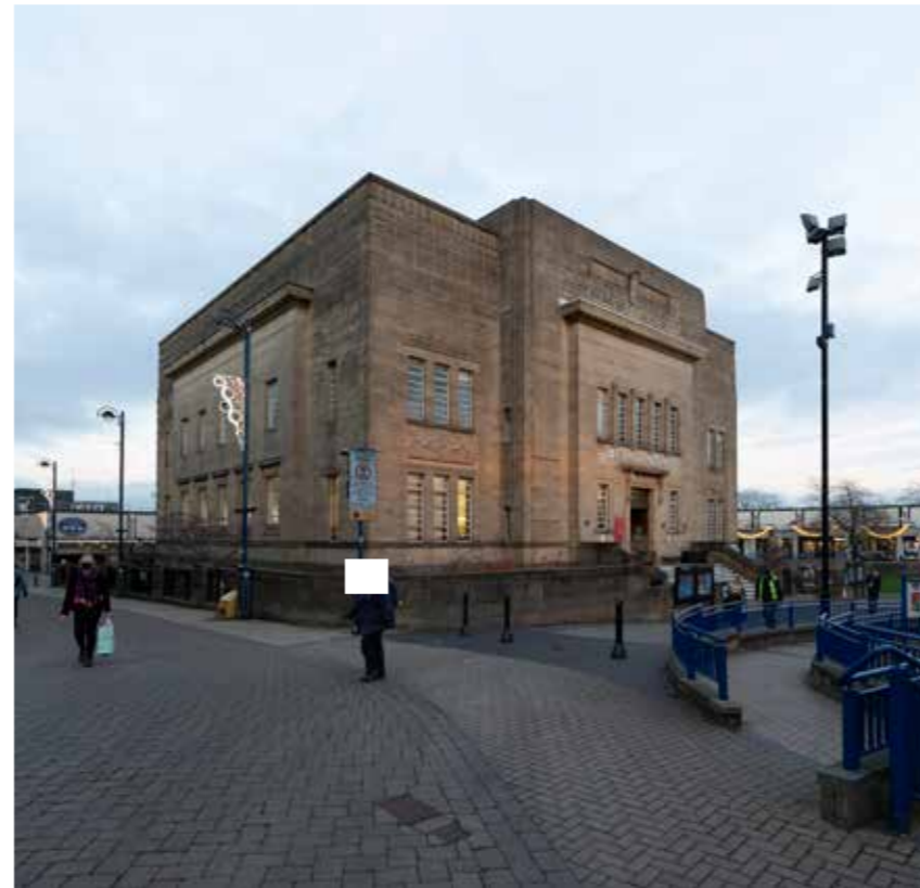
4.3.1 - Library and Art Gallery viewed from south-west
