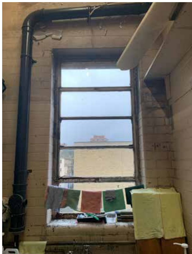
4.7.23 - Store / Service Room (Rm. 83)
