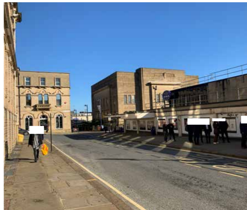
4.3.7 - View of building from Peel Street
