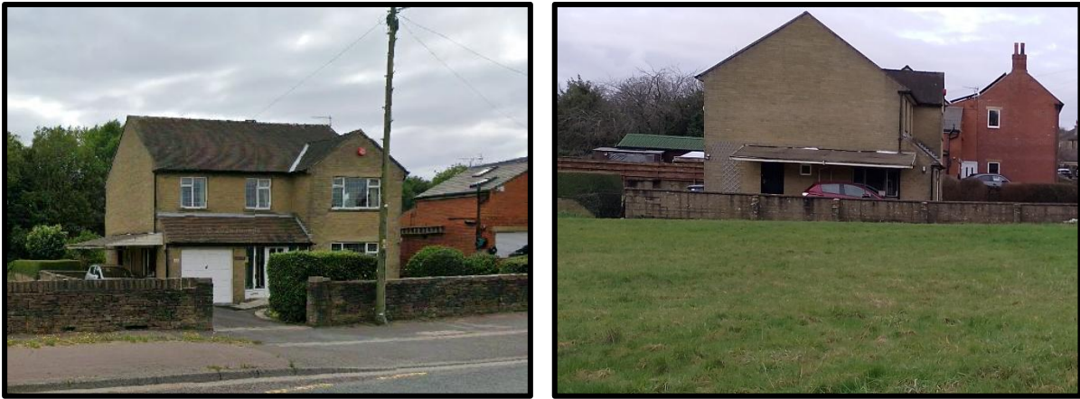
Figure 4: Building and Vegetated Garden
