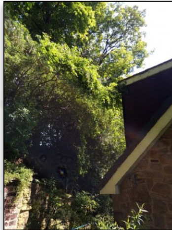
Image 5 - Showing T008 (l) branches in proximity to current building
