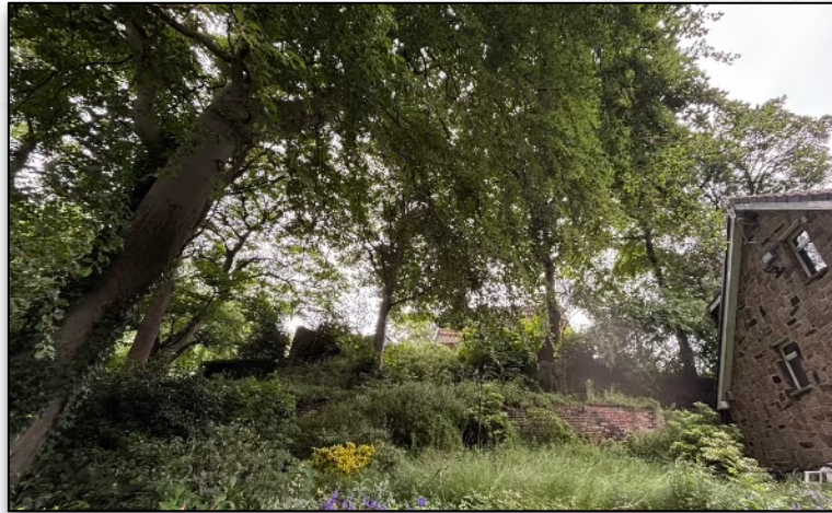
Image 2 - Showing T001, in proximity to main building with wide angle lens. Wall with high level soil change can be seen near the main building
