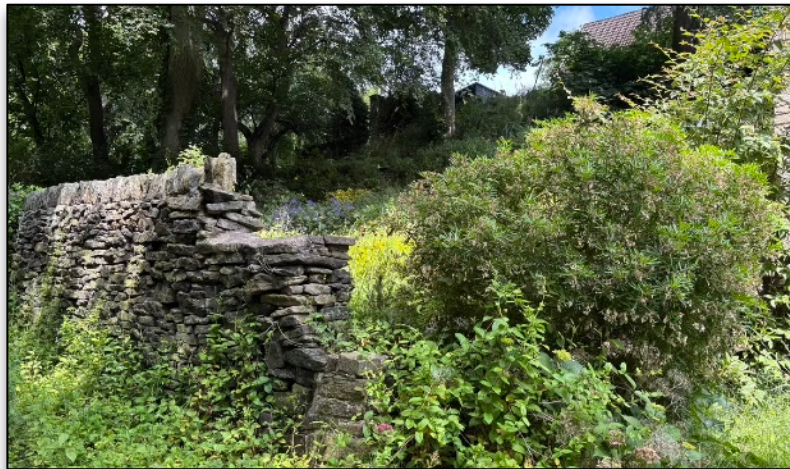
Image 4 - Showing front wall and small shrub that would likely serve as the site access
