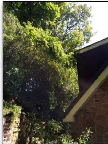
Image 5 - Showing T008 (I) branches in proximity to current building
