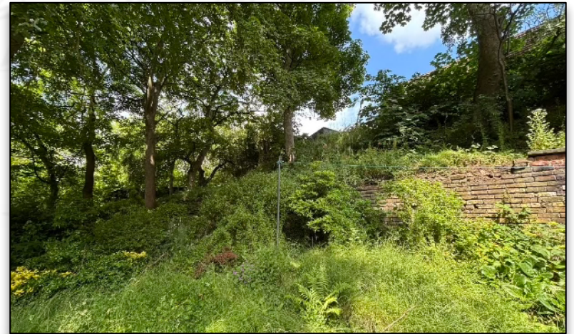
Image 3 - Showing high wall to rear of property, grading of R to L (E to W)/. T004 can be seen on the bank to the right of the image.
