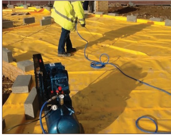
Figure A4.44 Air lance test, used to test the quality of welded seams along gas membrane joints (courtesy MEC Environmental Ltd)
