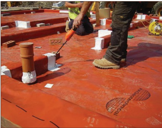
Figure A4.39 Scanning for leaks (courtesy PAGeotechnical Ltd)
