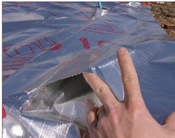
Figure A4.78 Gap in jointing over wall cavity big enough to insert fist (courtesy Smith Grant)
