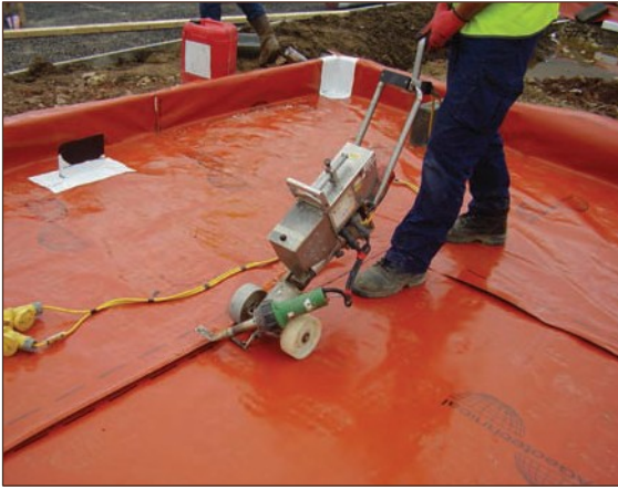
Figure A4.31 Extrusion welding (courtesy PAGeotechnical Ltd)
