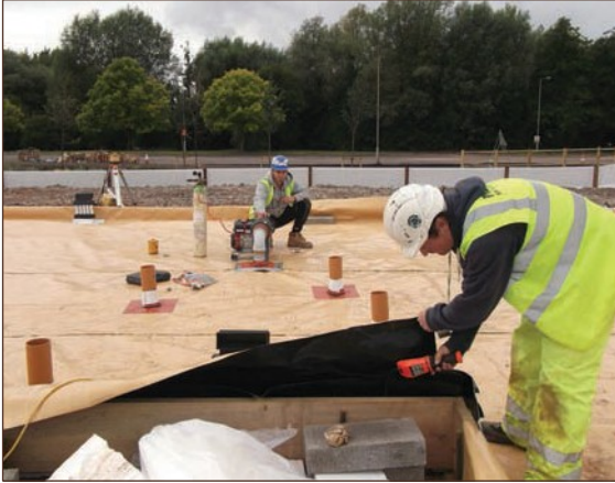
Figure A4.37 Tracer gas testing, whereby gas or smoke is applied under pressure beneath the installed gas membrane and detectors are used to screen for leaks above (courtesy NHBC)
