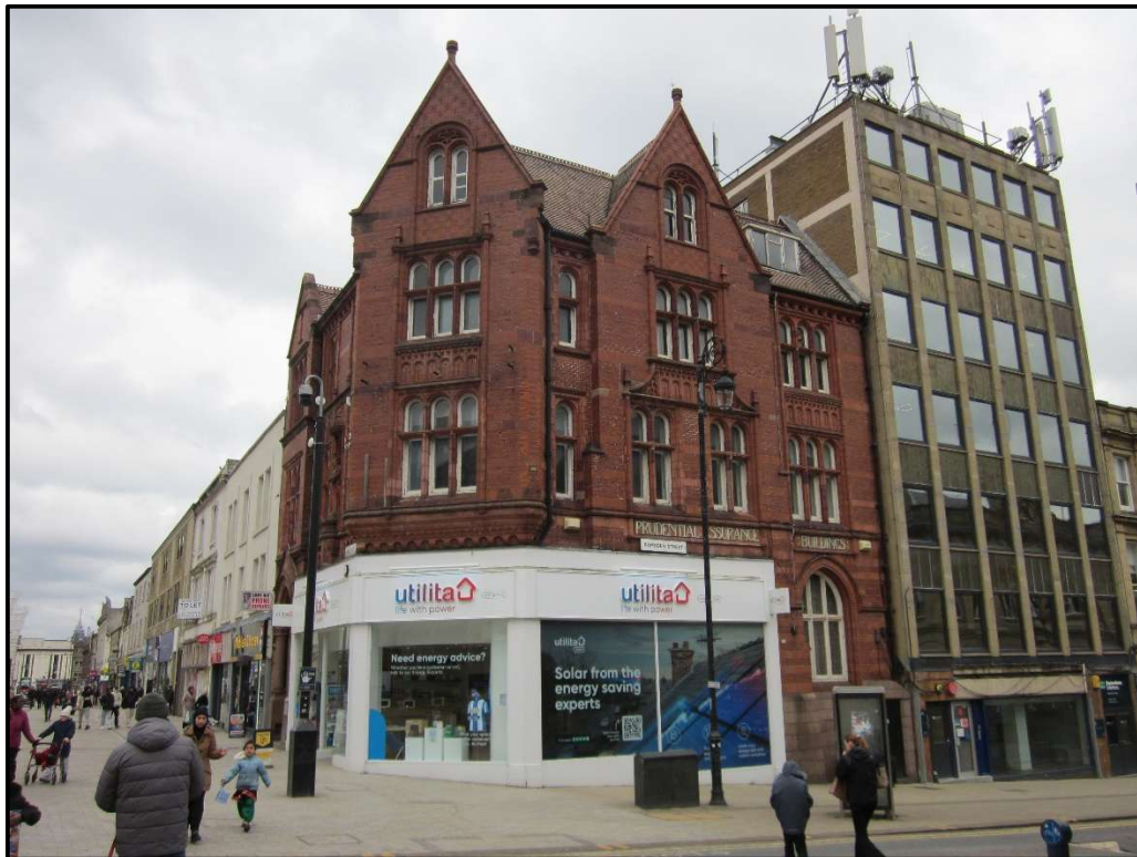
Photograph 1. Prudential House building at 69 – 71 New Street (looking North East)
