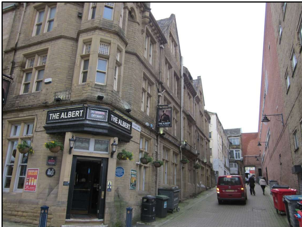
Photograph 6. The Albert public house at the junction of Albert Yard and Victoria Lane
