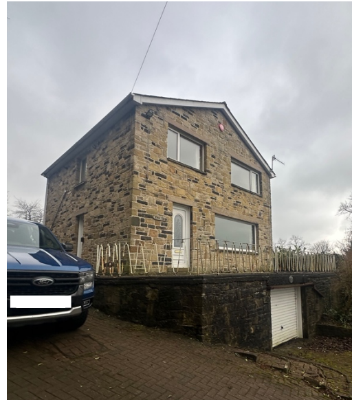
Figure 2 – Existing North Elevation
