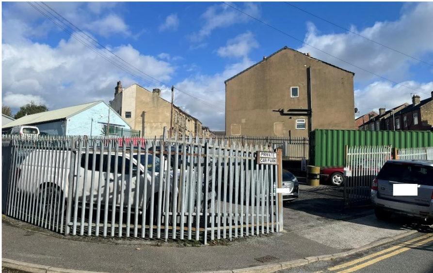
EXISTING SITE ENTRANCE FROM PEEL STREET
