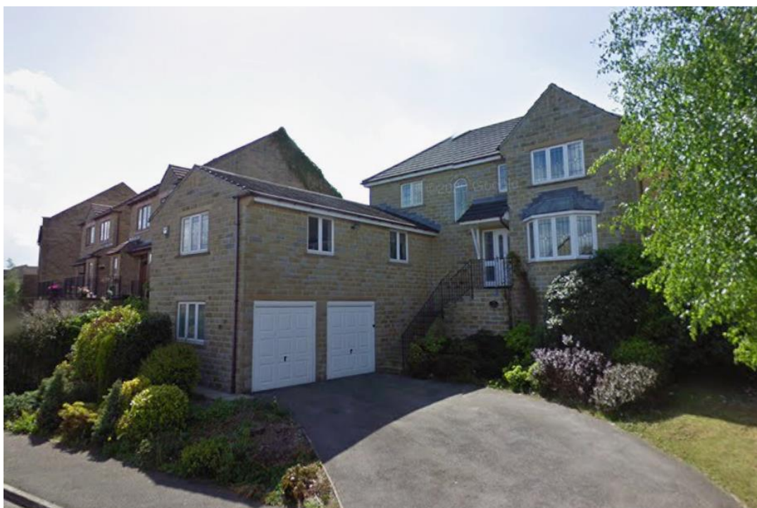
Image 2. – 112D Hawthorne Way Looking East Towards 130.
