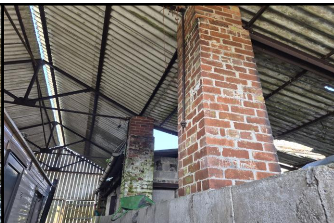
Photograph 8. Internal of Building 2
