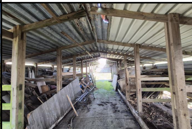
Photograph 6. Internal of Building 1
