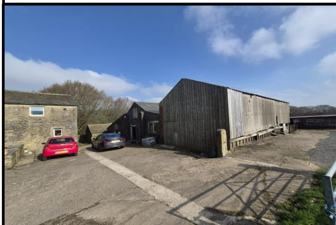
Photograph 3. Southwest corner of Building 2
