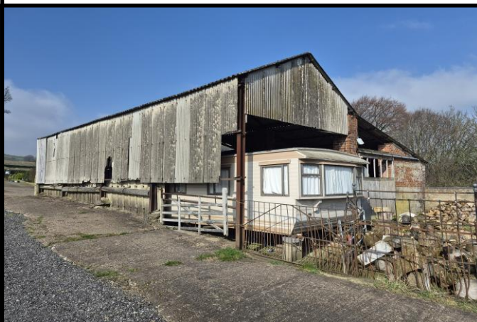
Photograph 4. Southeast corner of Building 2
