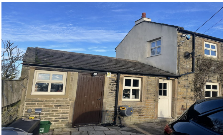
First Floor extension and front Porch to be built on top and to the front of existing building
