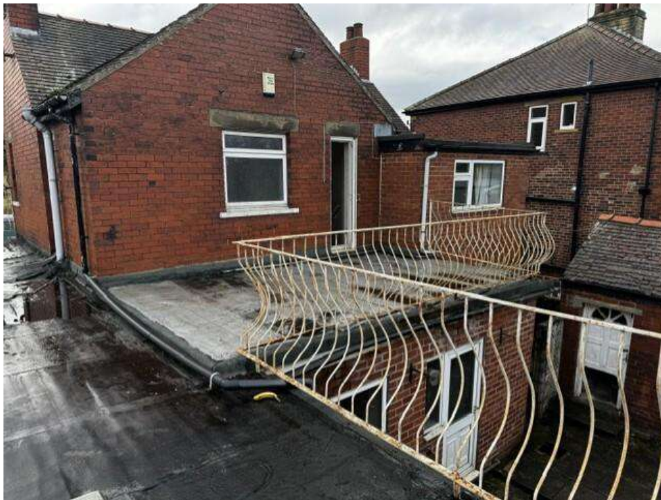
Door from House to Roof Terrace
