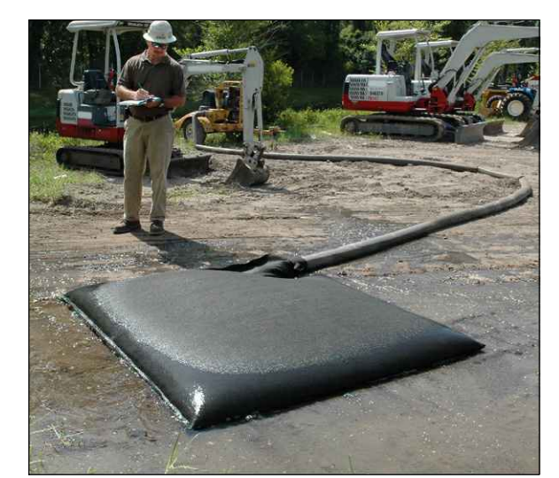
PHOTO OF DIRT BAG / SILT SOCK USAGE (NTS)
