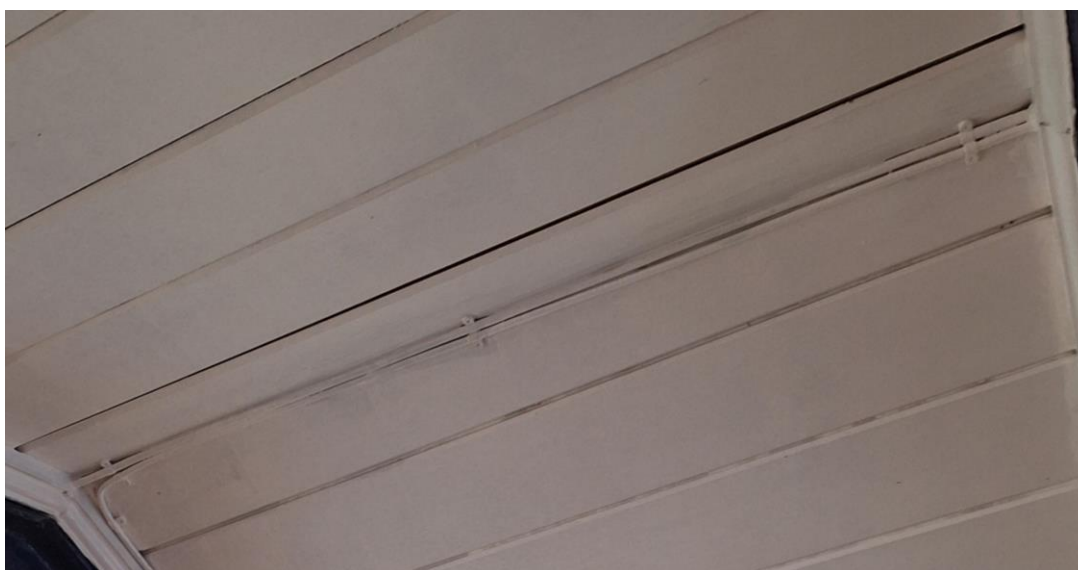
Insert 3-18 Existing cable fixed to the timber roof with cable clips
