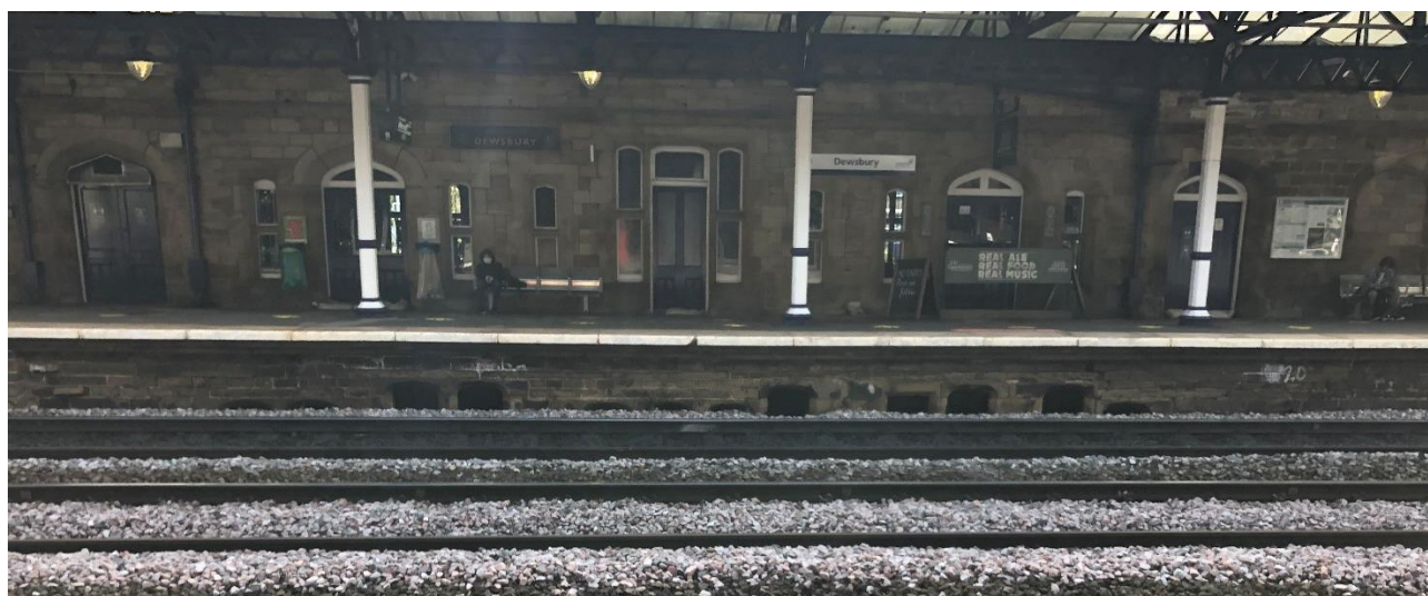
Insert 4-1 View from Platform 1 looking at the subway windows on the riser wall of Platform 2
