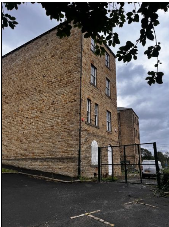
General view to the south west looking from site towards Rouse Mill Lane
