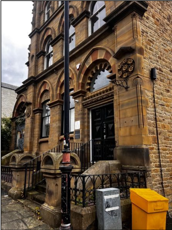
General view to the south west looking at site from Station Road
