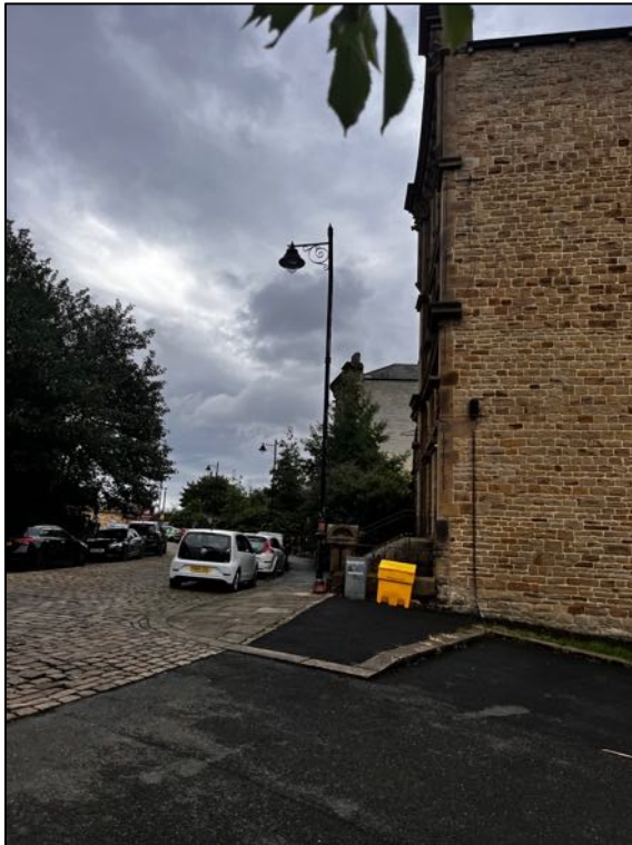
General view to the west looking at site from Station Road
