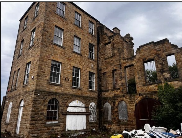
General view to the south west looking at site from Station Road
