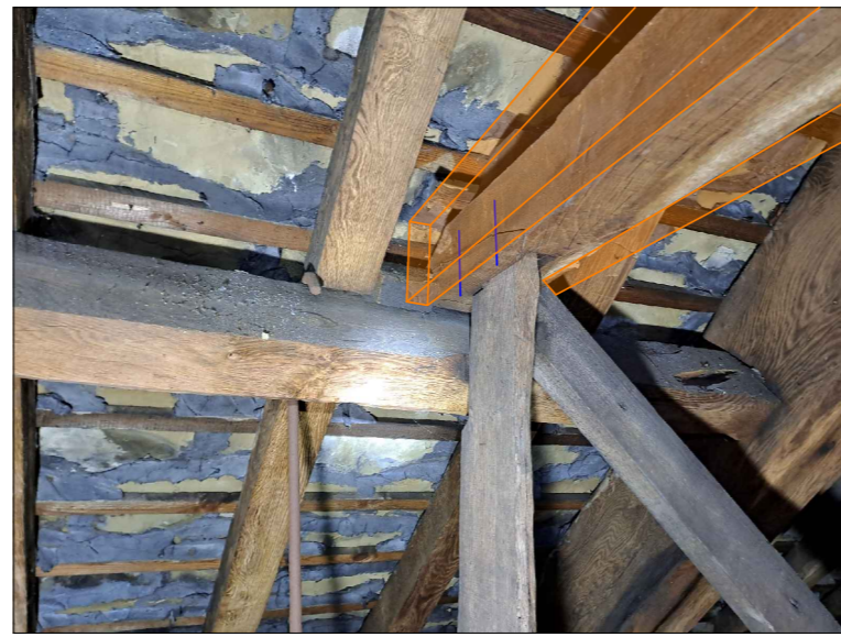
Infill splits and cracks with suitable timber resin the splits along the tie beams of trusses and ceiling beams.
