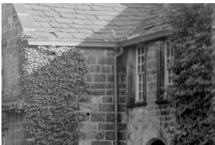
Photo c. 1900. Cast iron gutters and pipes with cast iron swan necks.
