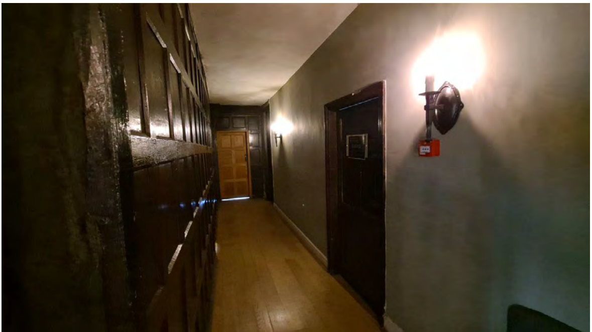
Photo 57: Corridor with toilets and access to Lady's Chamber
