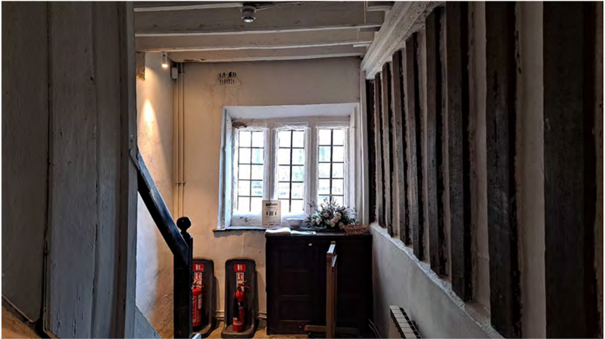
Photo 81: Corridor leading to back stairs looking south-east
