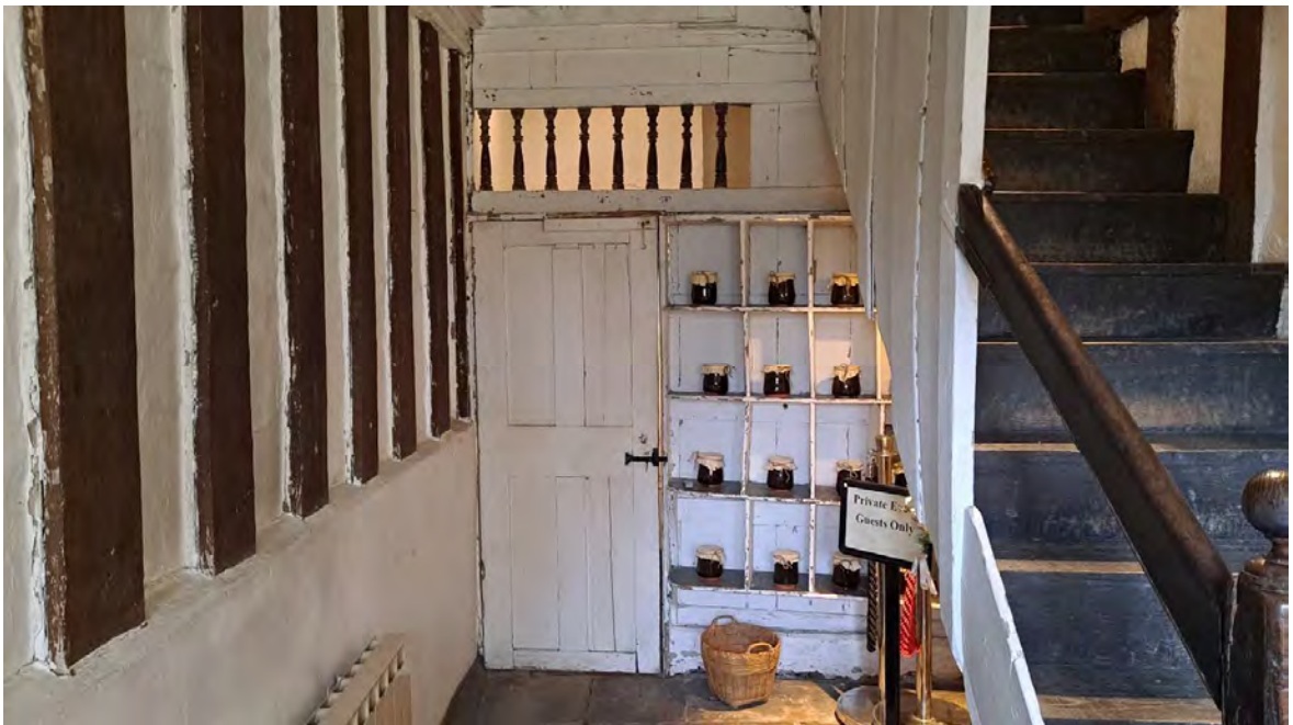
Photo 80: Back stairs and corridor looking north-west
