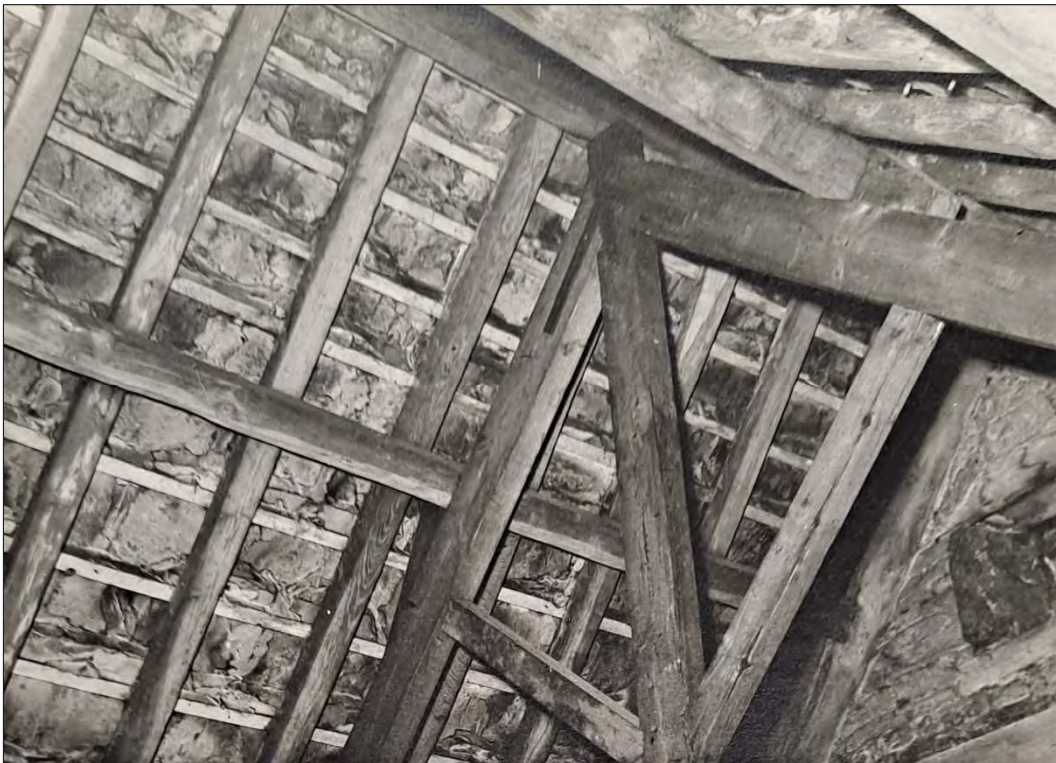
Figure 20: Exposed roof structure in the Kitchen Chamber
