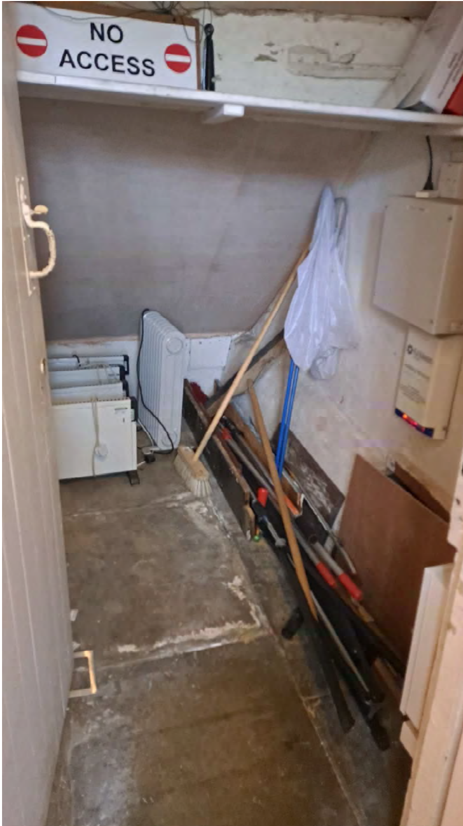
Photo 86: Possible former entrance to external cellar
