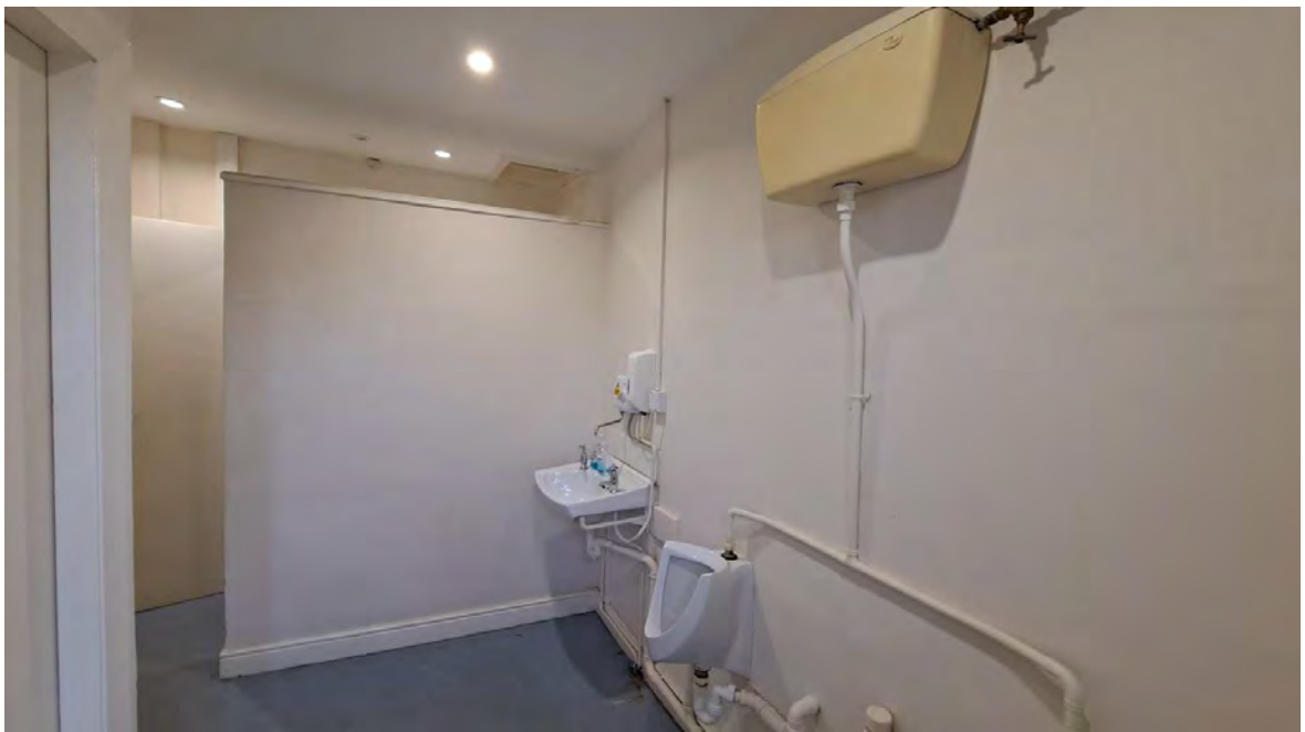
Photo 65: Internal partitions to gentlemens 'toilets
