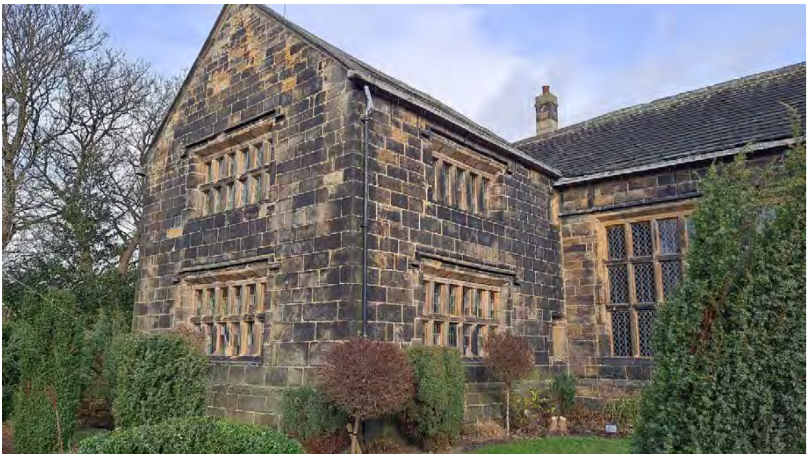
Photo 12: The west wing from the south
