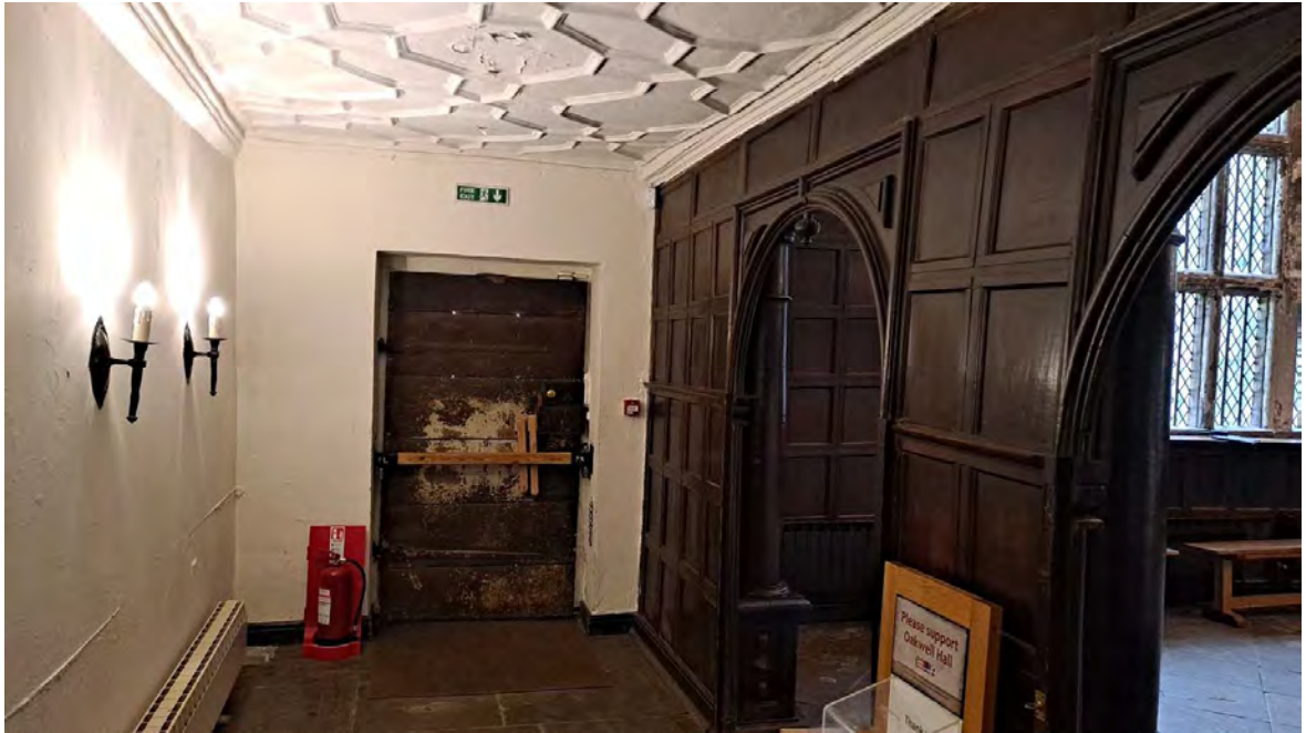
Photo 29: Main doorway in screened passage looking south-west
