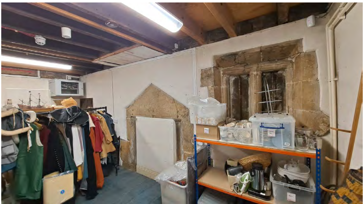
Photo 46: Former Pantry with sealed fireplace and blocked window
