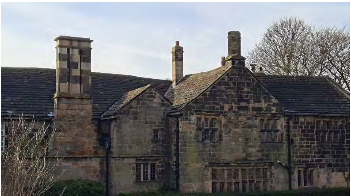
Photo 24: Rear elevation from north-east with stair turret to left centre
