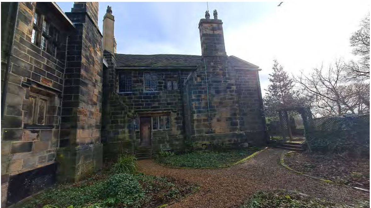
Photo 18: The north-west elevation of the west wing
