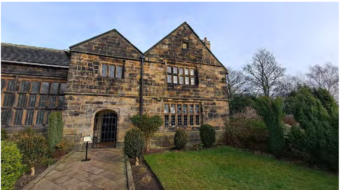
Photo 14: The east wing and the gabled porch
