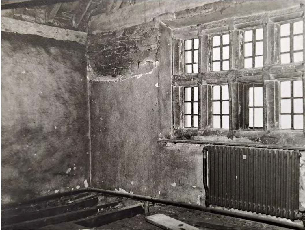
Figure 19: Restoration work in the Kitchen Chamber
