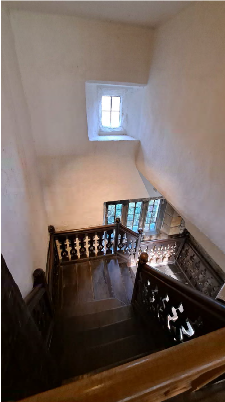
Photo 67: The original staircase in the stair turret
