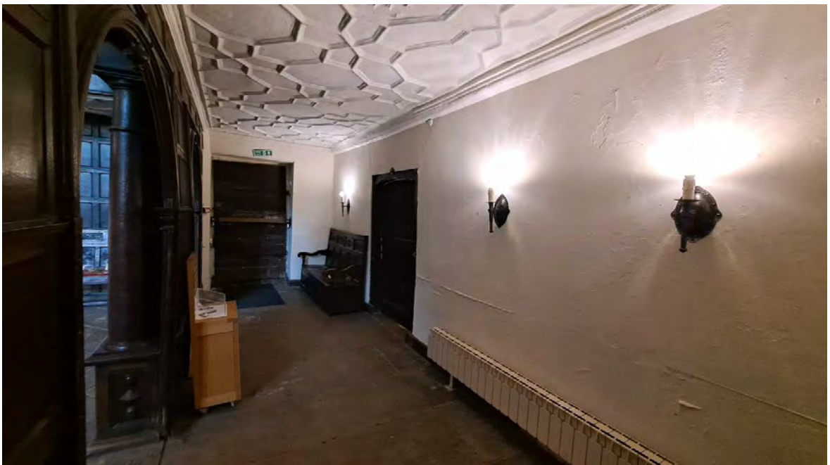
Photo 28: Screened passage looking north-east with doorway to east wing to centre
