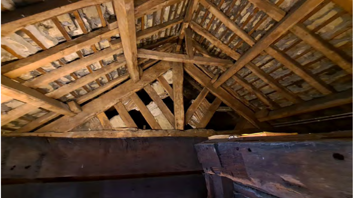
Photo 75: Detail of roof structure from Porch Chamber looking north-west
