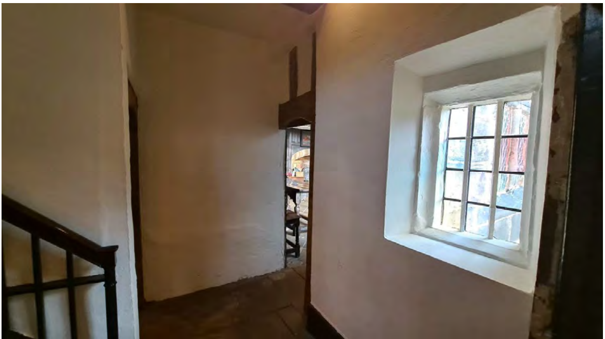
Photo 36: Lobby to the west of the Hall
