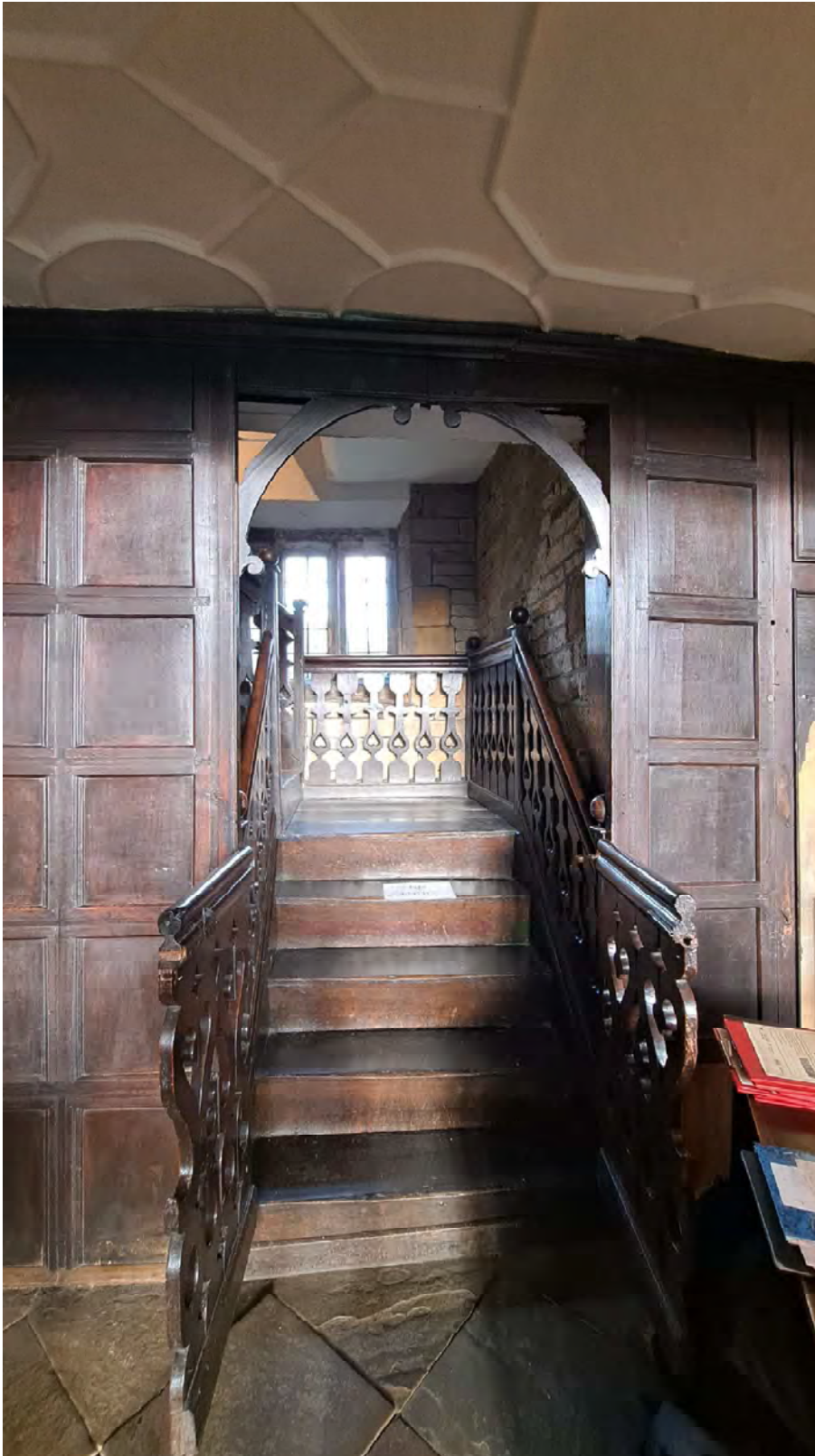
Photo 47: Original staircase with dog gates
