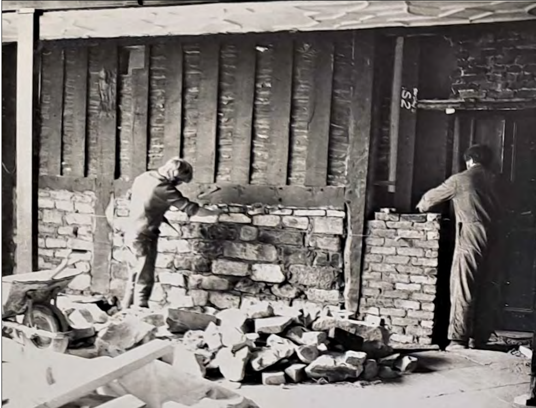
Figure 16: Renovation work to the Great Hall
