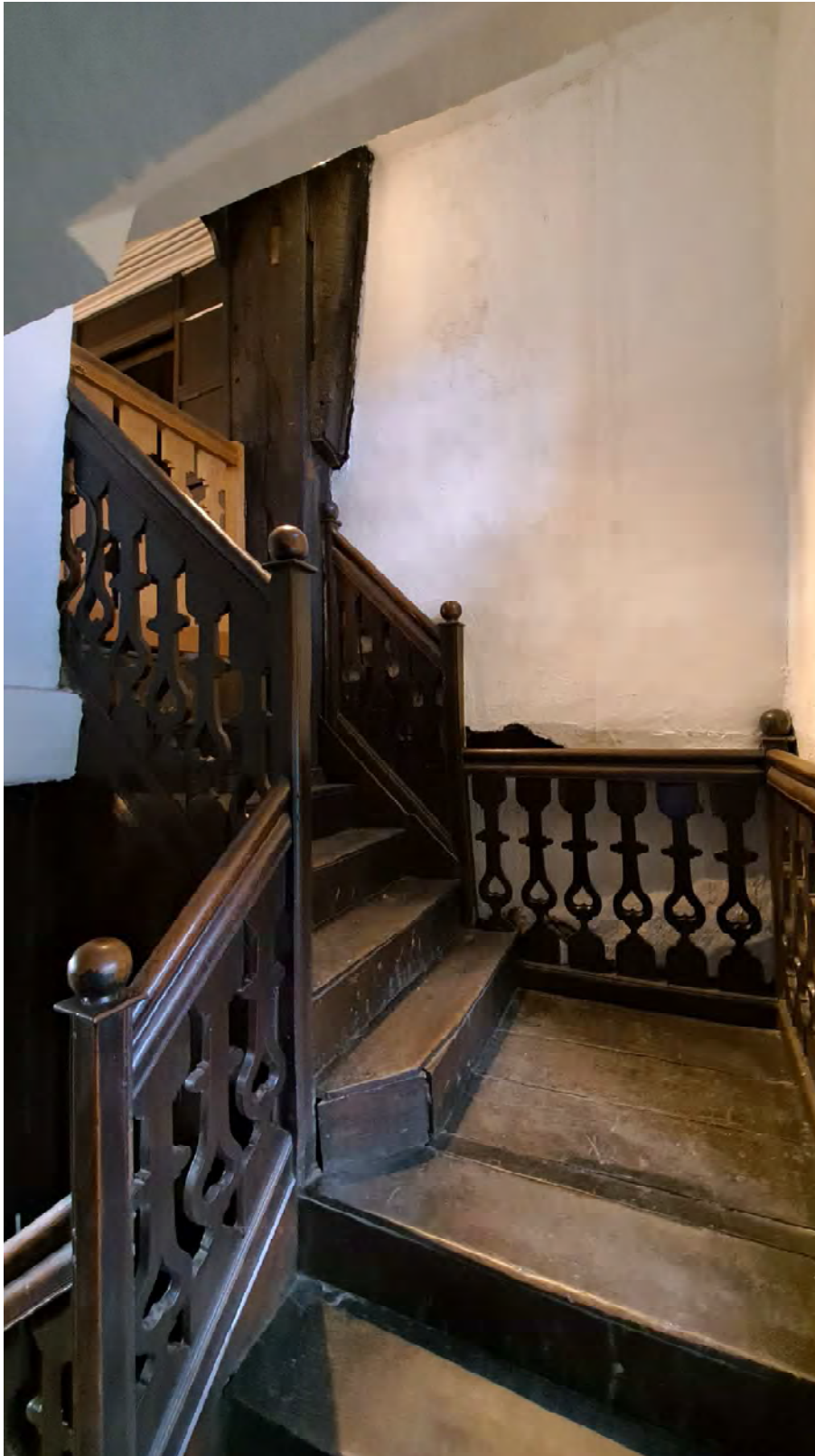
Photo 48: Detail of original staircase
