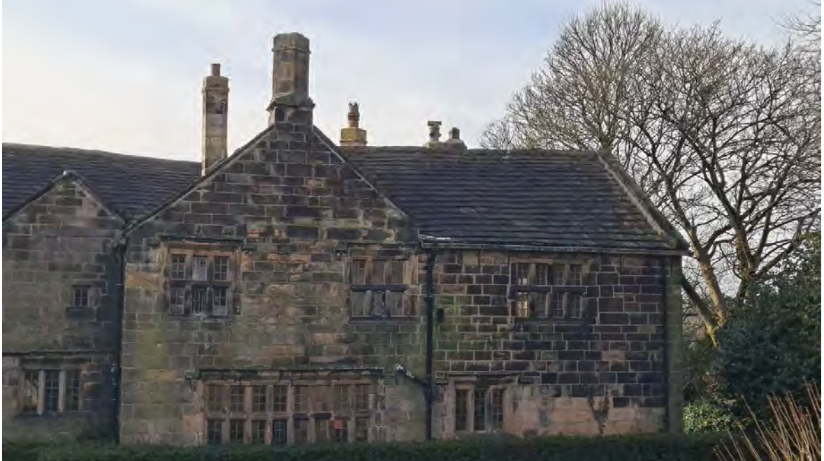
Photo 23: The rear of the west wing with gabled dairy wing to right
