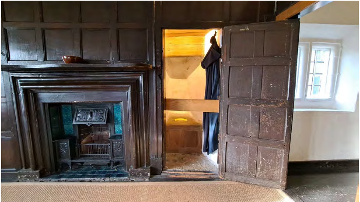
Photo 54: Concealed privy or garderobe in Great Parlour Chamber
