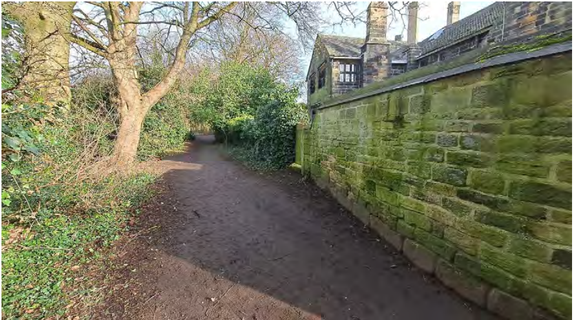
Photo 4: Footpath to the west of the Hall showing boundary wall
