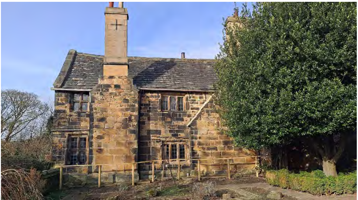
Photo 16: The south-east elevation
