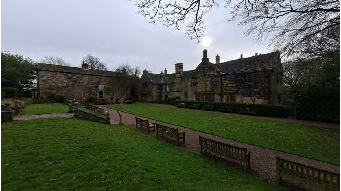
Photo 21: Oblique view from the north
