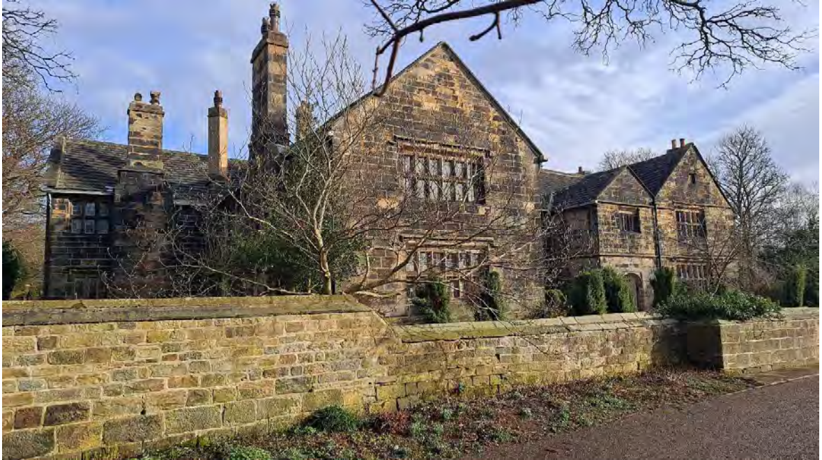
Photo 9: The Hall from the west
