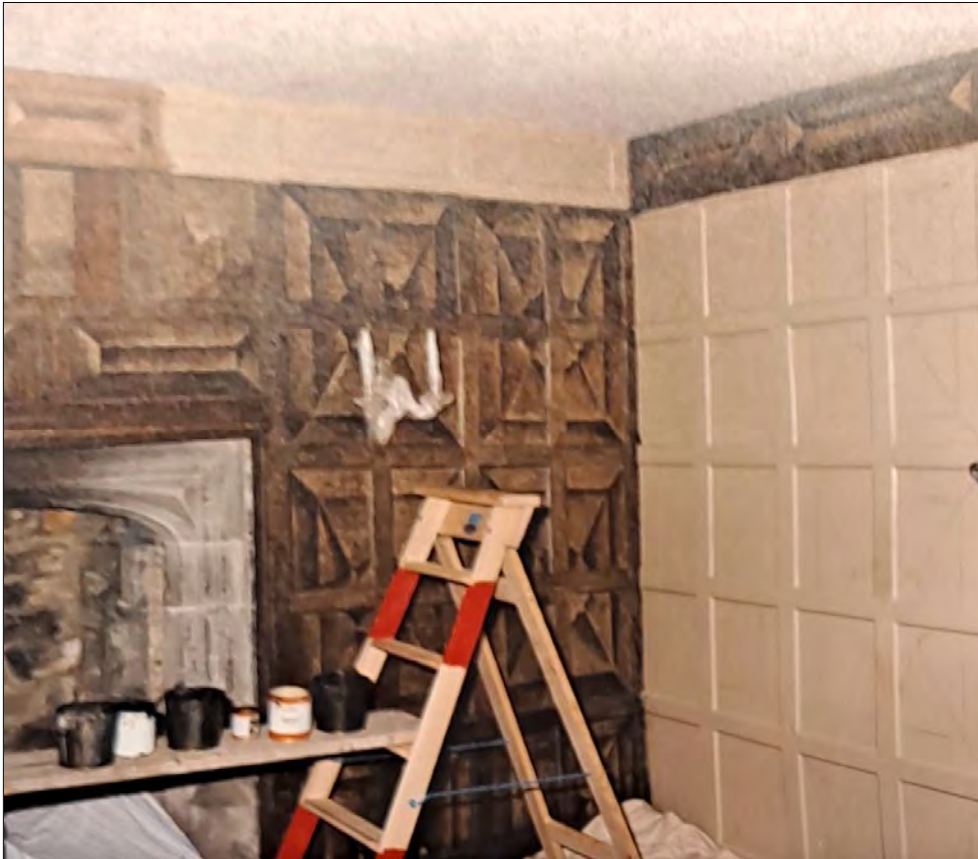
Figure 23: Restoration work to Great Parlour Chamber
