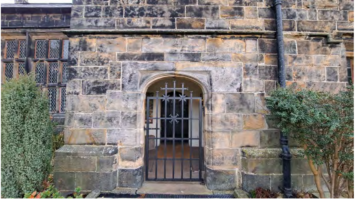
Photo 27: Detail to main entrance (south-west)
