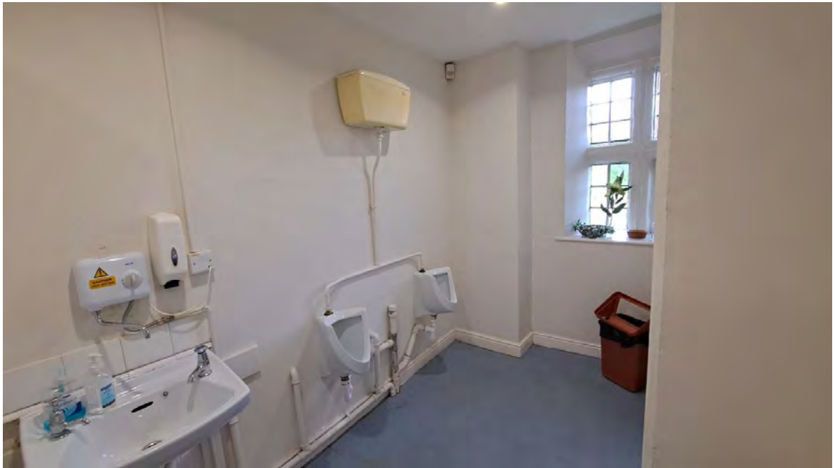
Photo 64: Interior view of gentlemens 'toilets
