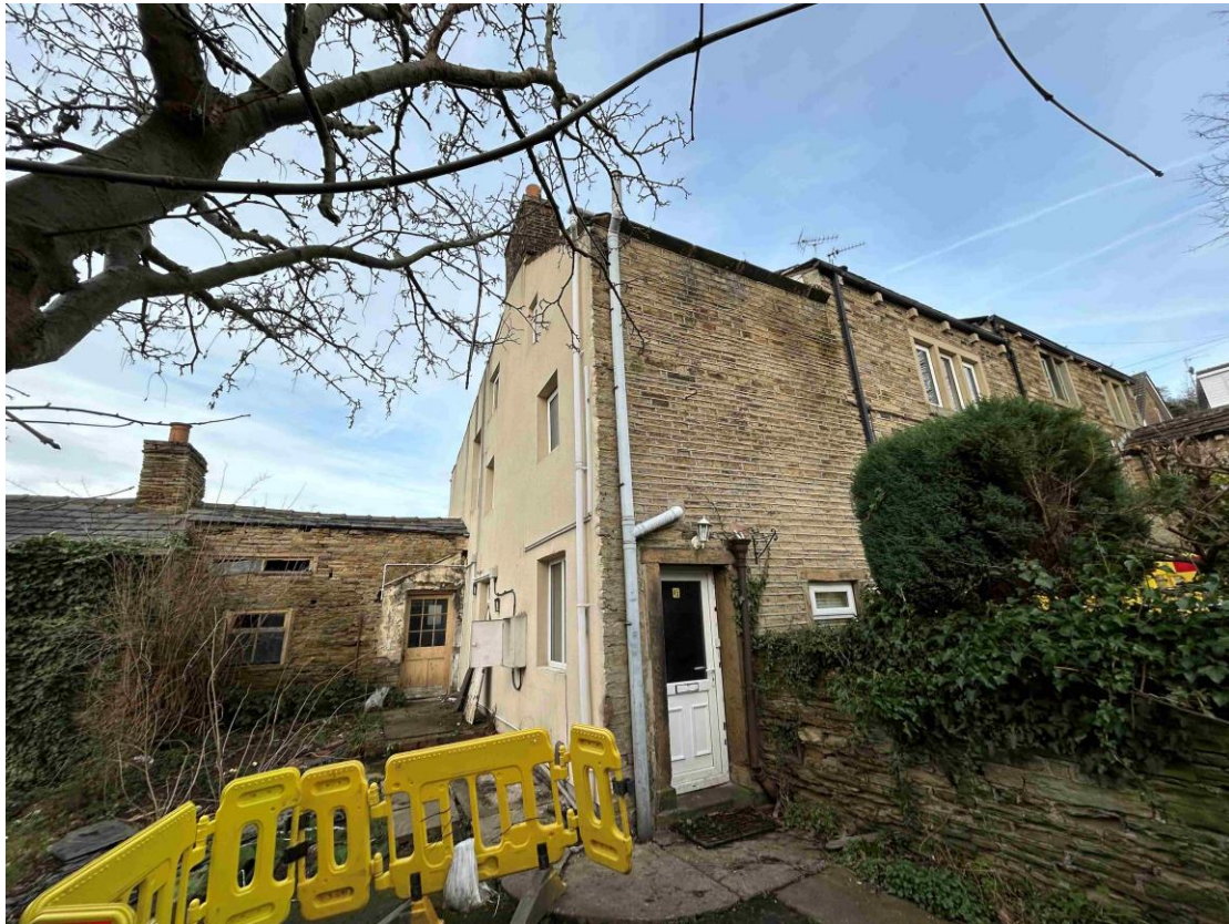
Photograph 8 – 45 Fenay Bridge Road
