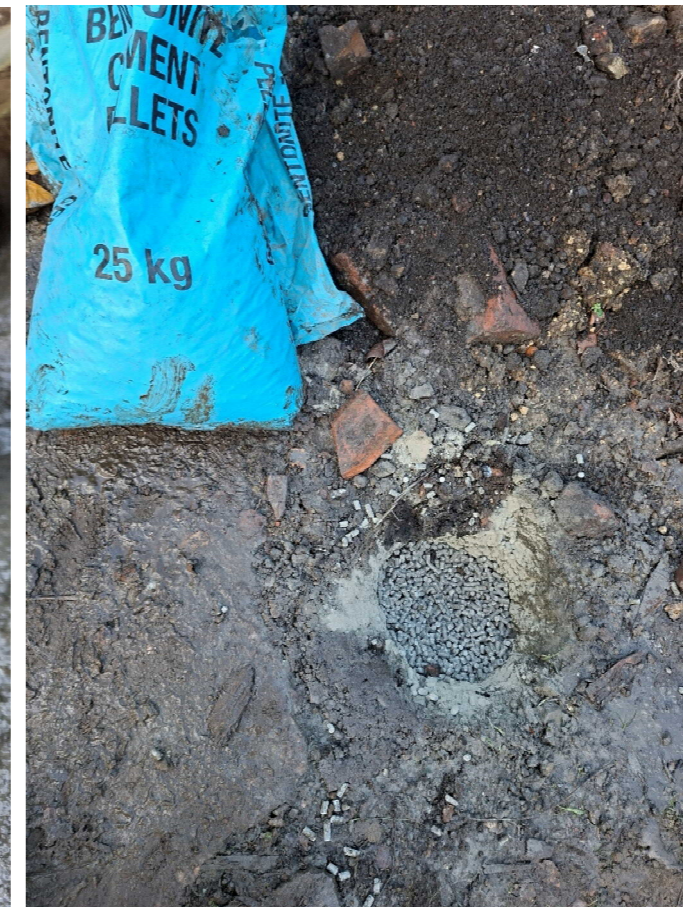
^^^ Photograph 4: Backfilling/sealing of R0101
