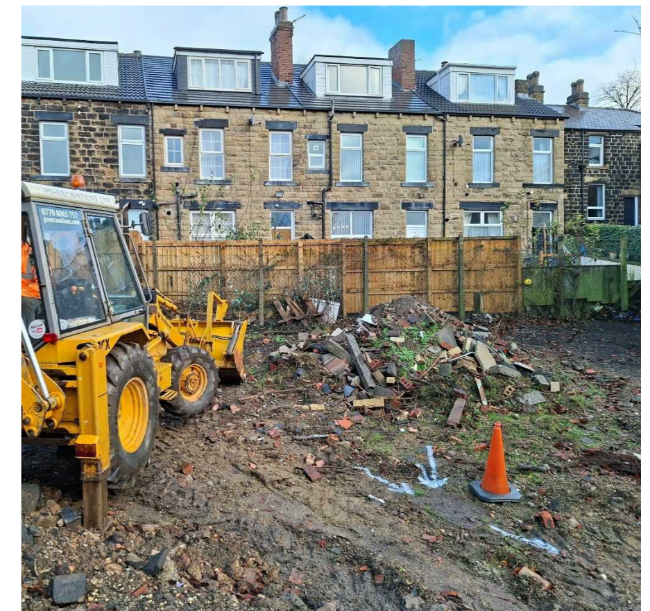
^^^ Photograph 3: Approximate alignment of drainage infrastructure within the central portion of the Site restricting access for investigation
