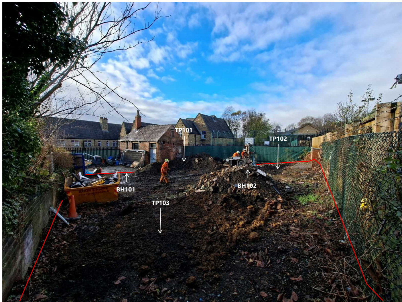
^^^ Photograph 1: General arrangement of the Site (looking south-west)
