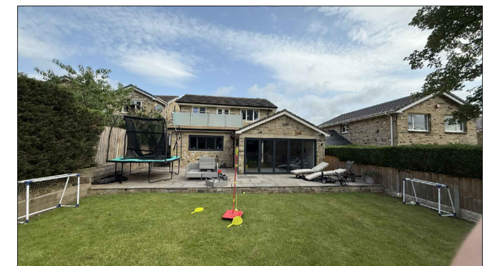
Rear Elevation Photograph As Existing
