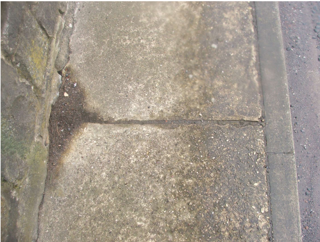
Typical formed contraction joint in concrete verge.
