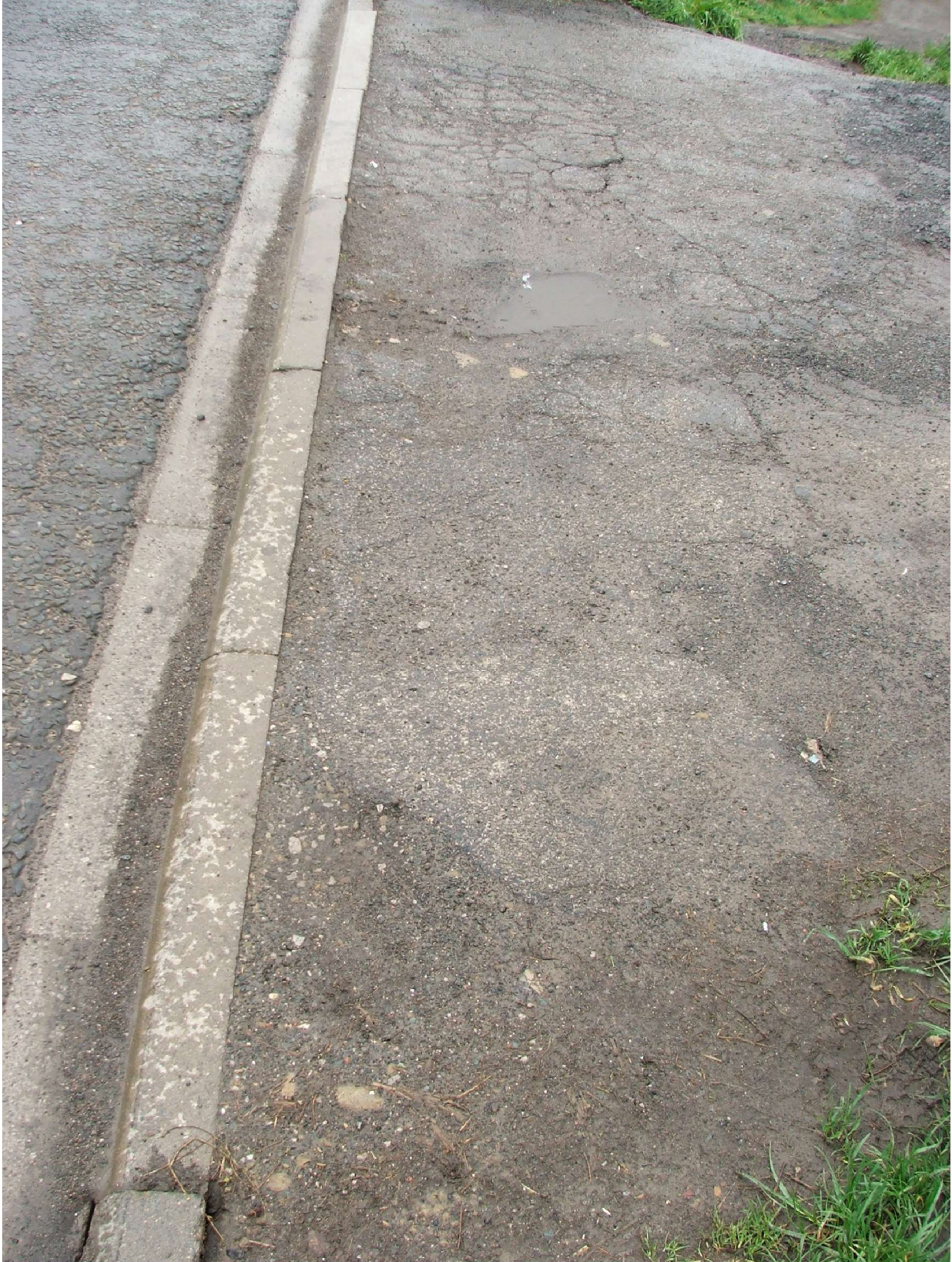
Dropped bull nose kerb across existing site access
