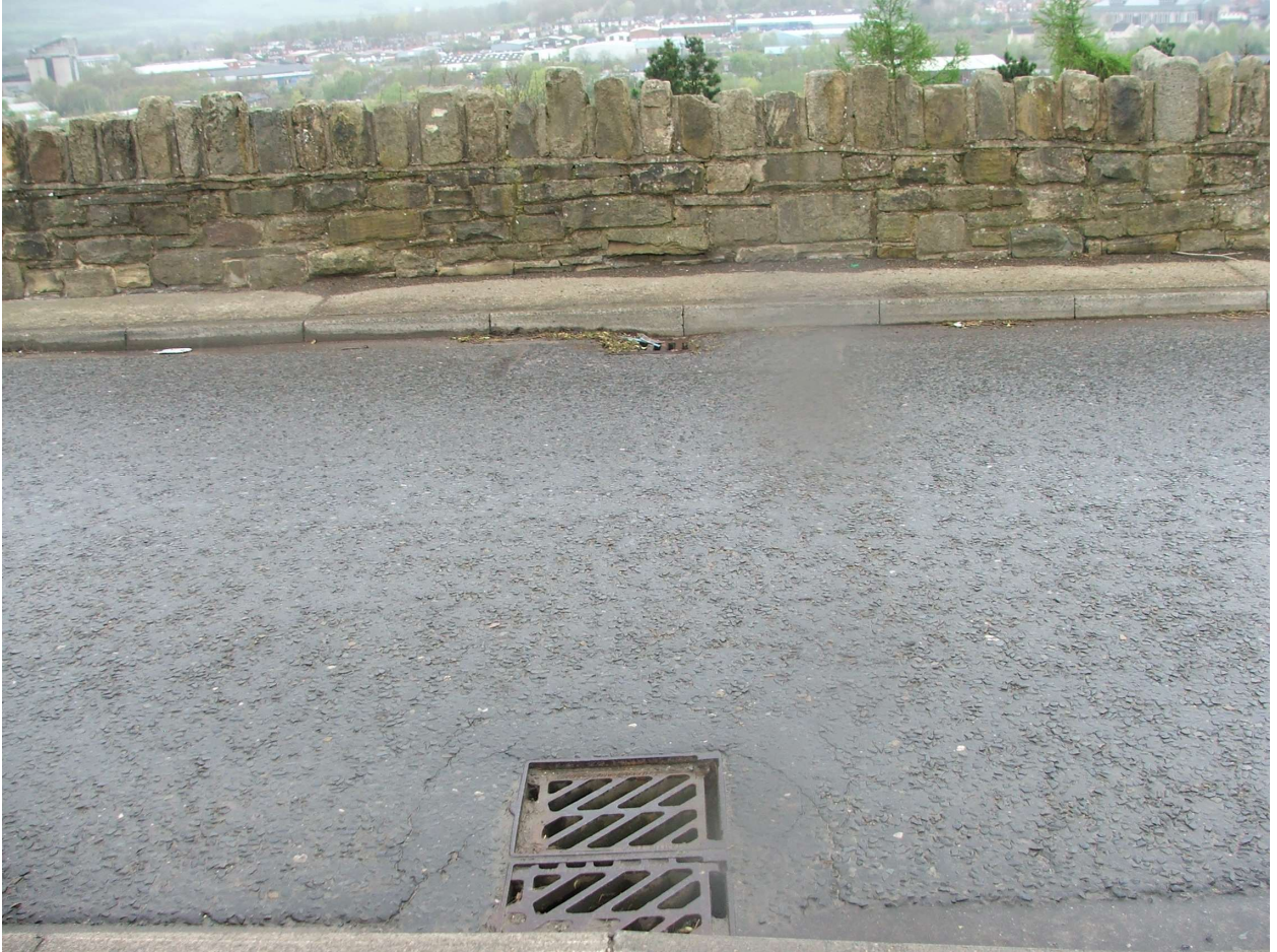
Highway drainage gullies
