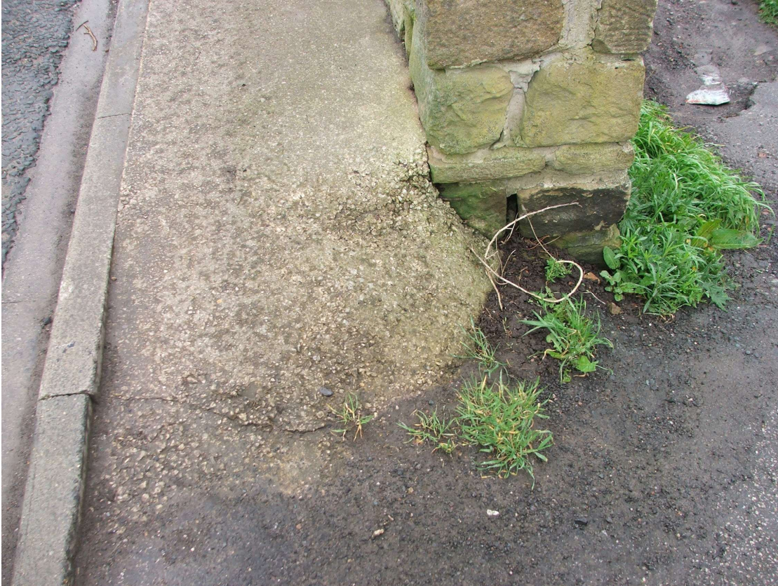
Start of concrete verge.
