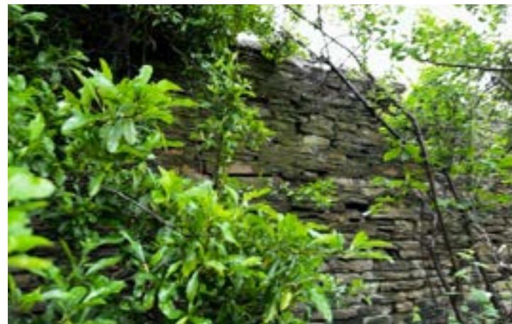
Image 6: Built linear feature (drystone wall)
