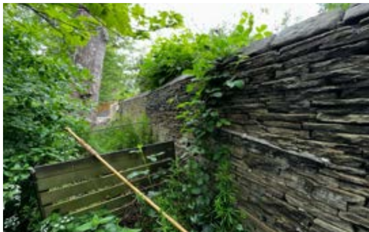
Image 5: Built linear feature (drystone wall)
