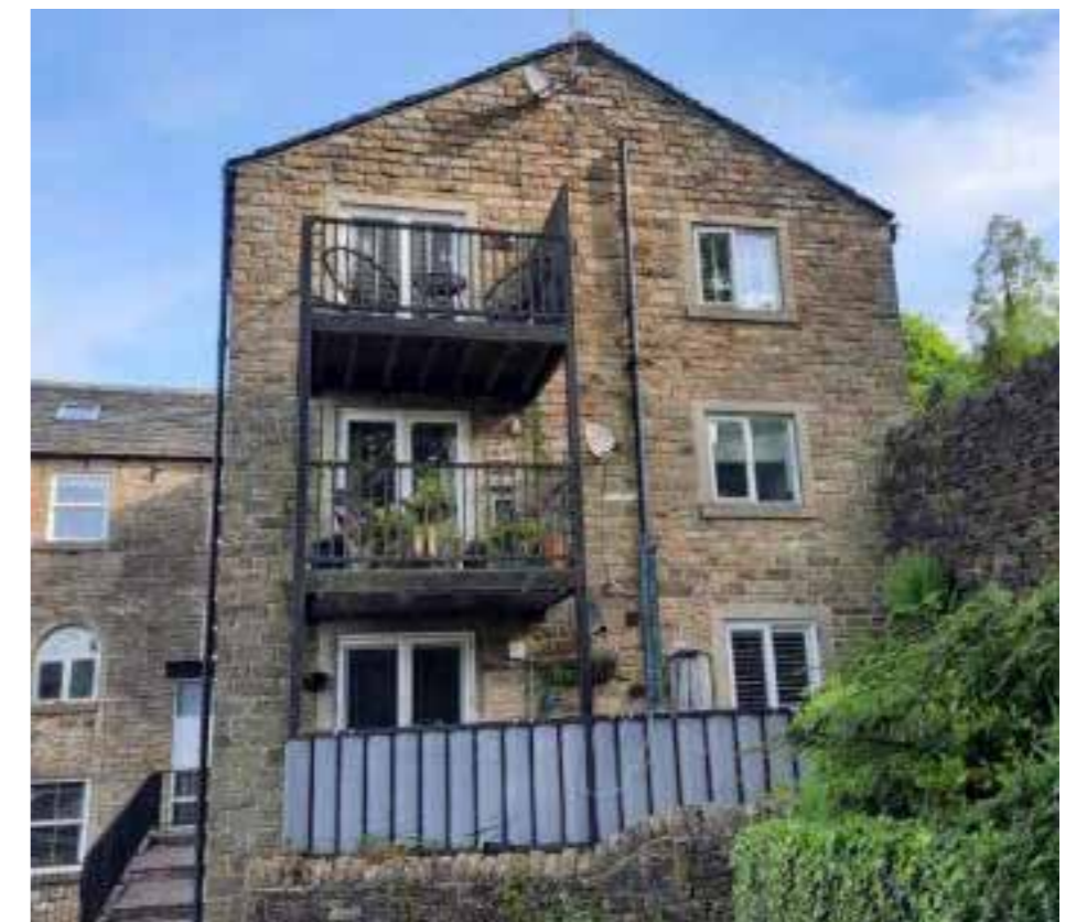
South Elevation - 116 Underbank.
