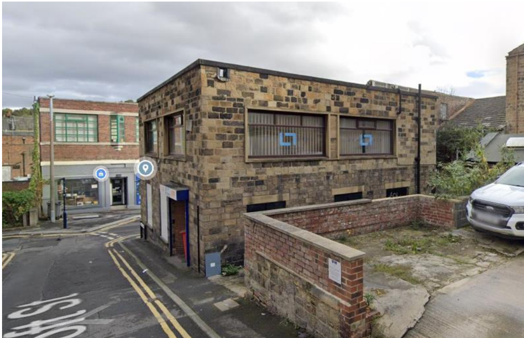
2.5 Above: Image shows the side and rear elevation of the building with access to rear yard area provided from Croft Street.
