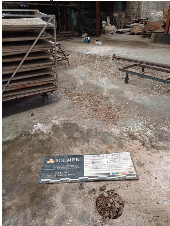
Figure 12: BH09 Location (backfilled)
