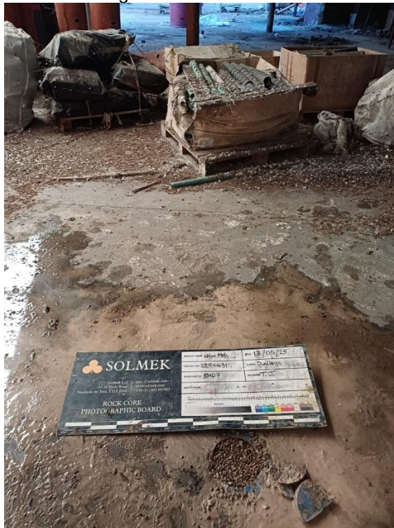
Figure 10: BH07 Location (backfilled)
