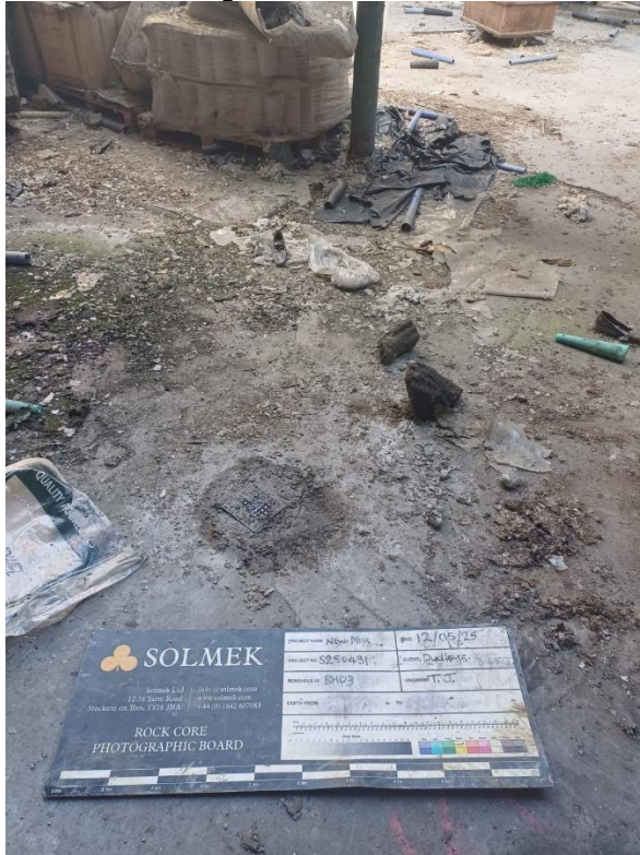
Figure 6: BH03 location (following completion/installation)
