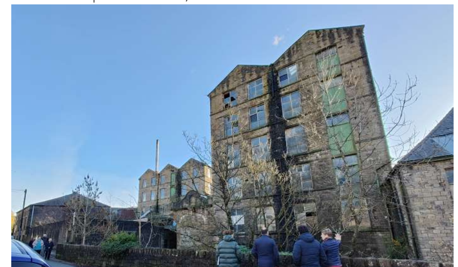
View of New Mills
