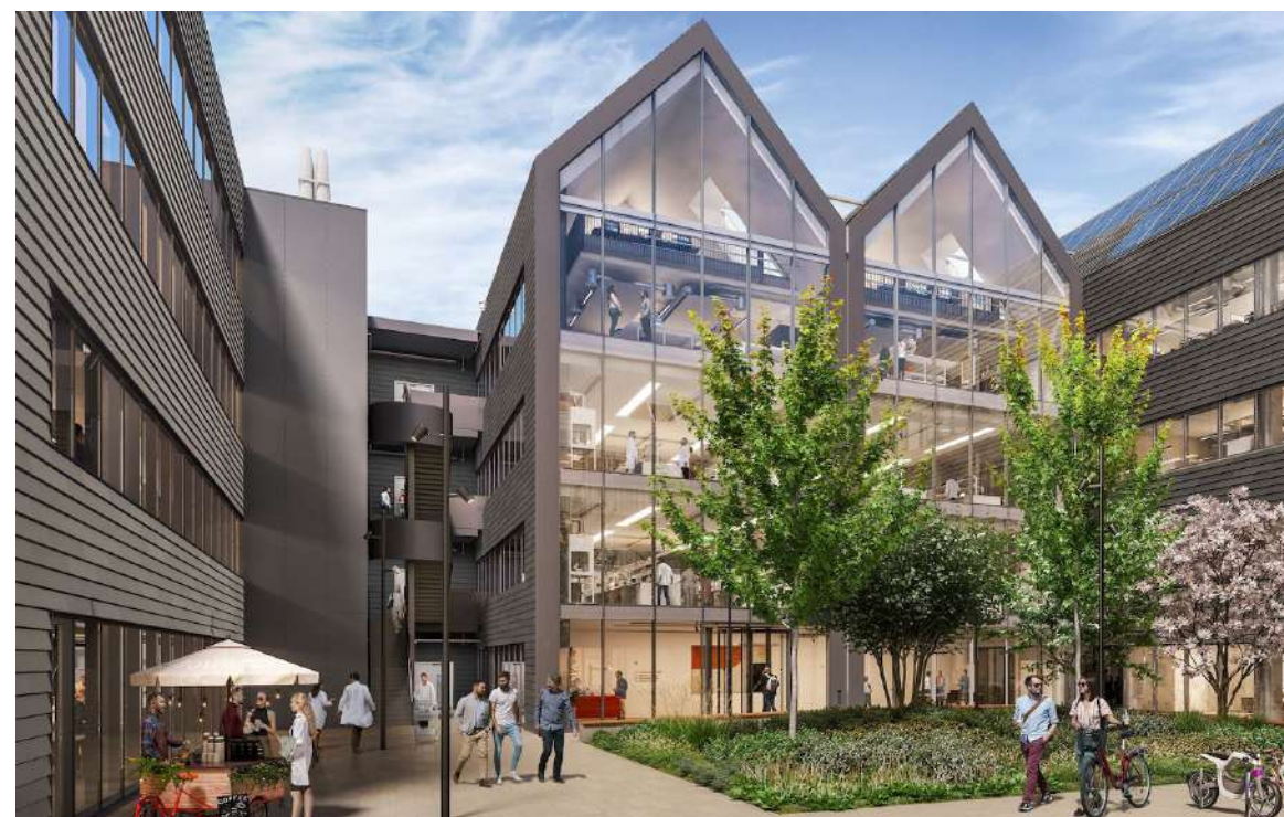
1 & 2 Fallaize Street, Oxford North - Oxford
