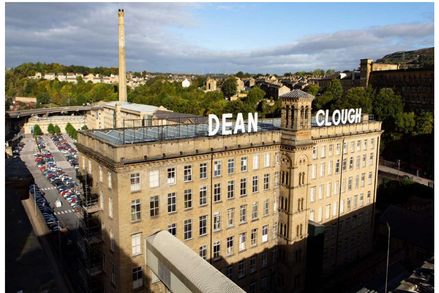
Dean Clough Mill, Huddersfield
