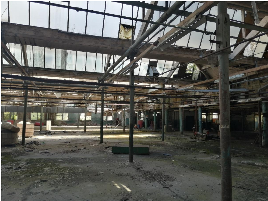
Figure 16 Interior of the large single storey mills.
