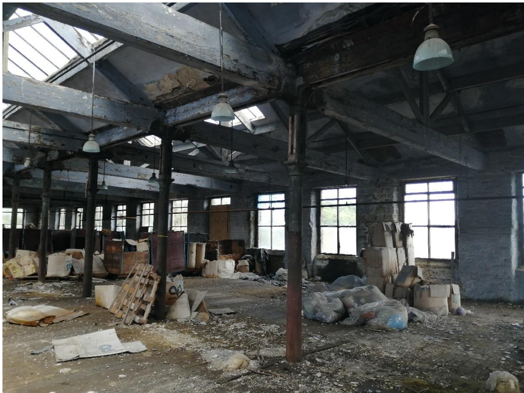
Figure 18 Top floor of Building A.
