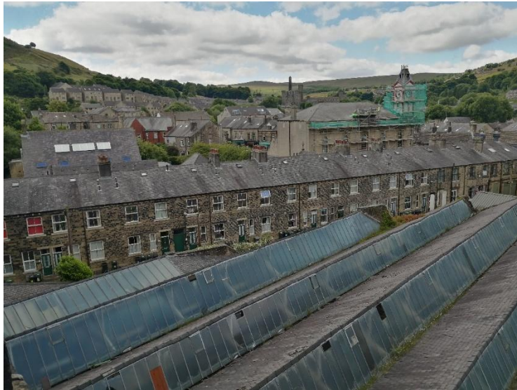
Figure 3 Looking down towards the low-level mill buildings and Derby Terrace.
