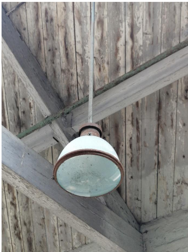
Figure 23 Historic services remain in variable conditions.
