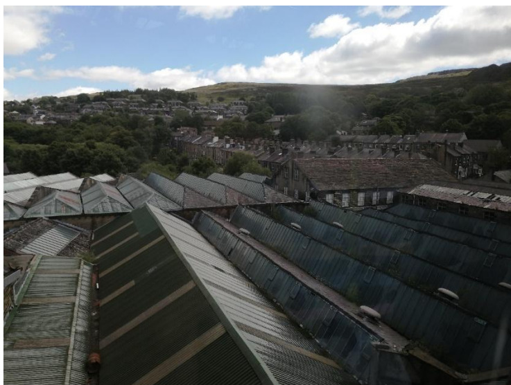
Figure 5 Looking across the low-level development to the East.
