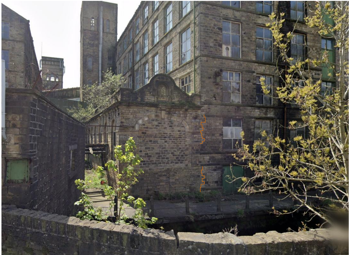
Figure 33 Photograph showing the joint in the built fabric
