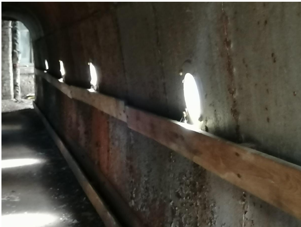
Figure 21 Interior of a high-level tunnel.
