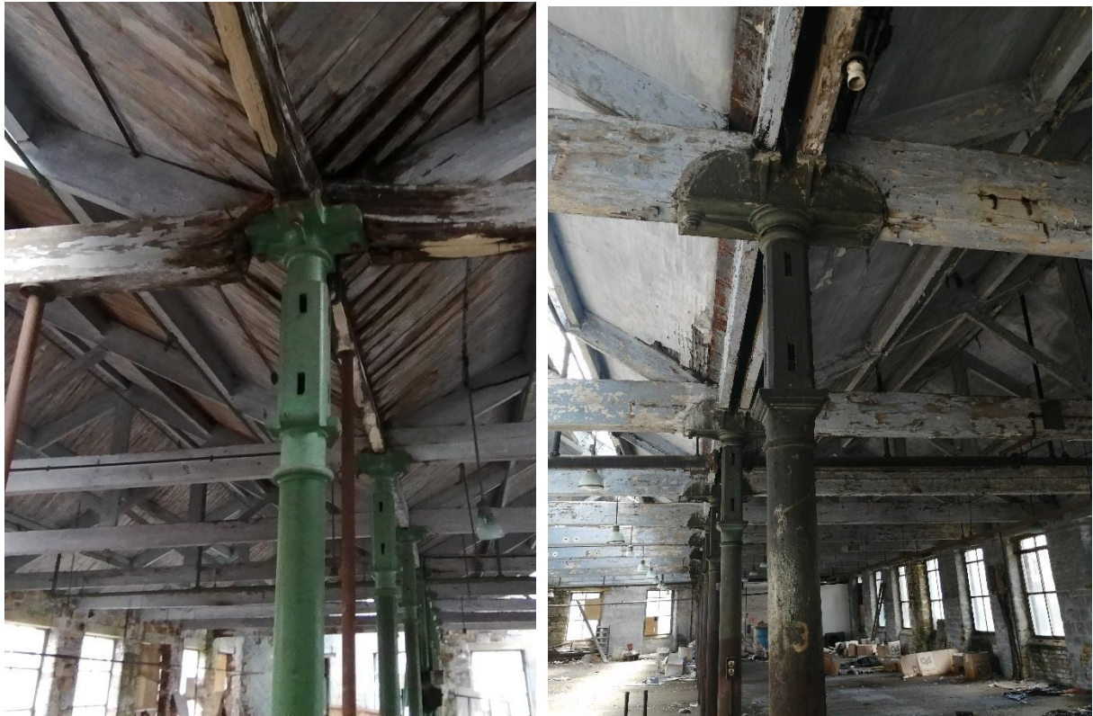
Figure 20 Iron columns support the timber floor and roof structures.
