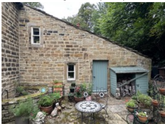
East elevation – catslide roof to the rear
