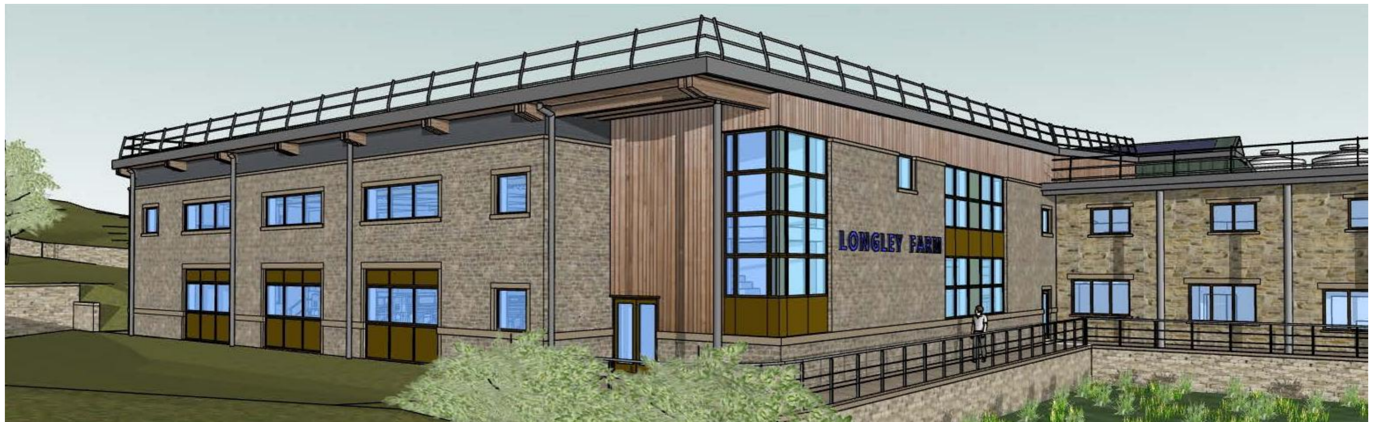
Image showing use of timber cladding on the north elevation beneath overhanging eaves on the new extension
