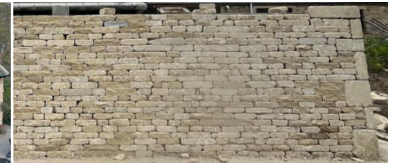
Coursed dry stone walling to dam wall (Crosland Moor Quarry)
