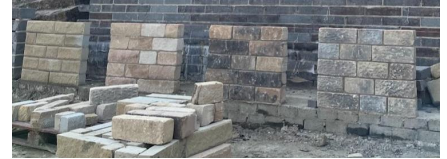
Sample Stone Panels on Site
