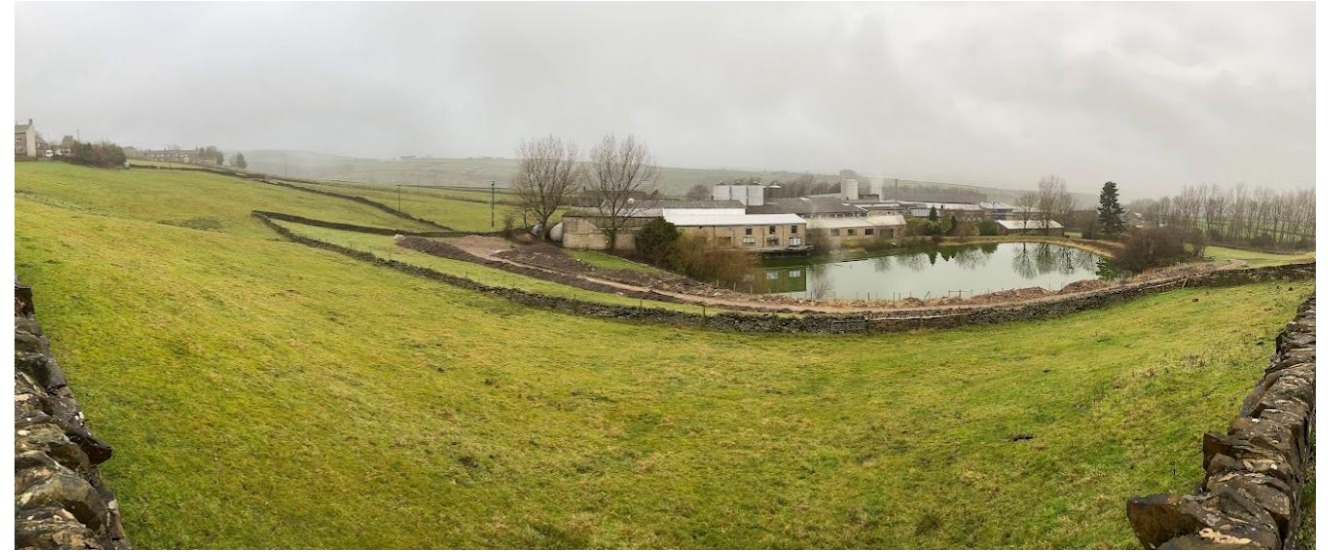
Longley Farm proposed site and Existing Dairy seen from Dunford Road (Bent Farm is visible on the left)
