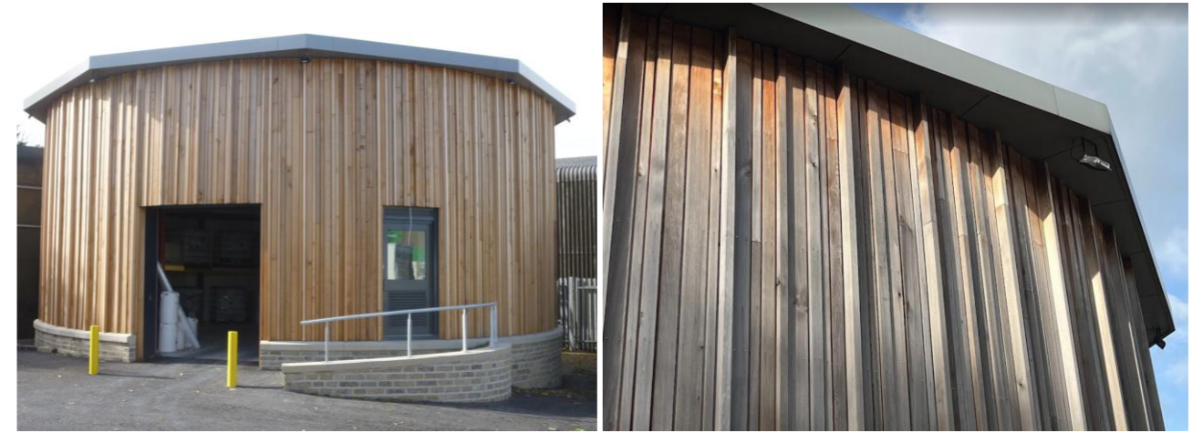
Converted Water Tank Clad in Cedar Cladding
