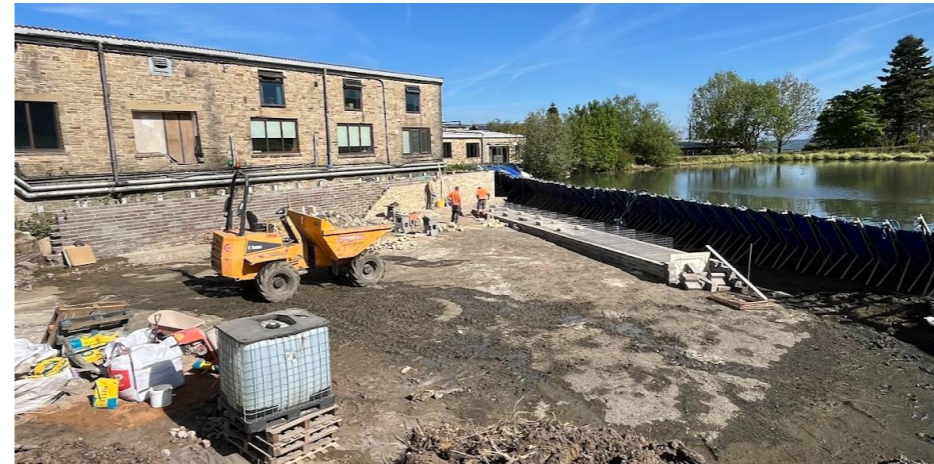
Temporary dam formed in order to repair existing dairy wall
