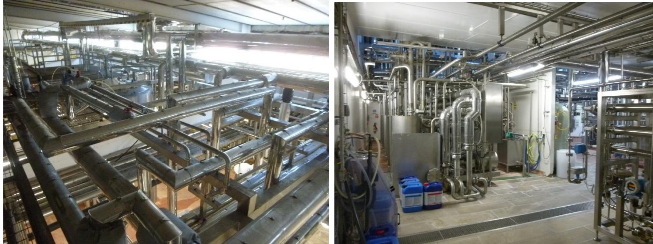
Photos showing existing cramped dairy services
