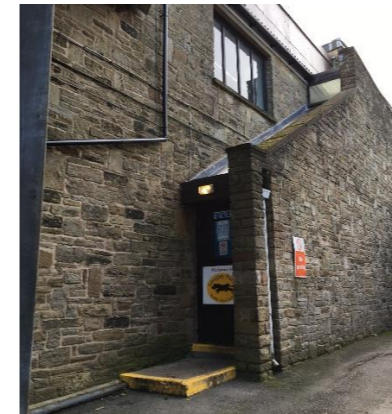
Existing Entrance with redundant stair
