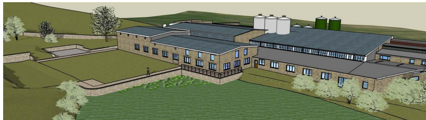
Birds Eye View of the Existing Dairy
