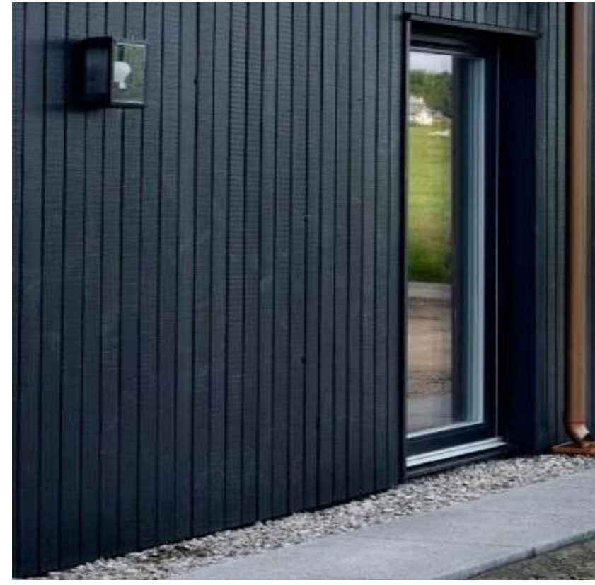
Black Vertical Slatted Timber Cladding
