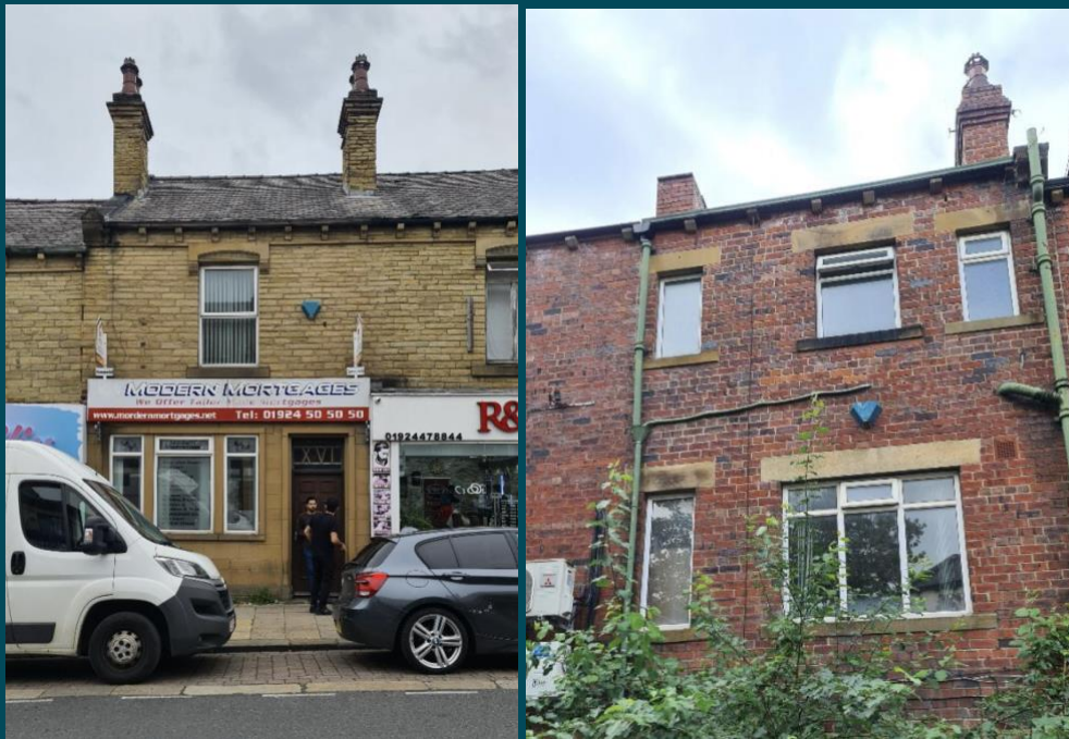
Fig. 3 – Existing Site Photo (front and rear elevations)
