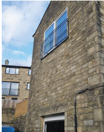
Figure 1: The Juliet balcony of the Site in the foreground with the similar designed Juliet and balustrade to 119A Woodhead Road in the background
