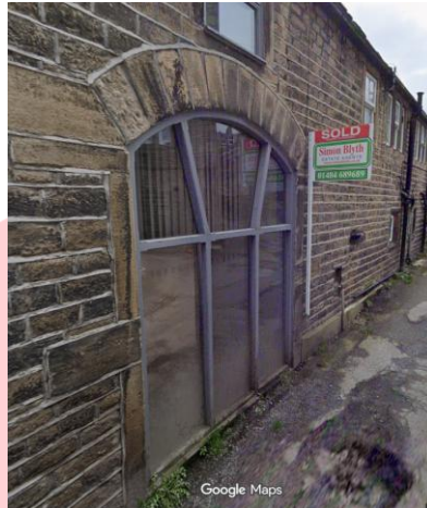
Figure 4: Floor to ceiling opening at 3 Water Street (image sourced from Google Maps)
