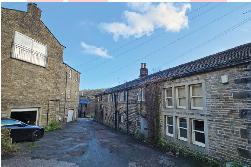
Figure 6: Photograph showing the stepped topography between the Site and 1a Water Street
