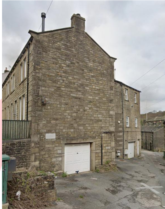
Figure 5: Side Elevation of the Site prior to the installation of the patio doors and balustrade (image sourced from Google Maps from survey dated April 2023)
