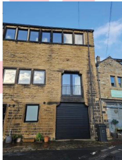
Figure 3: Photograph of the rear elevation of 119a Woodhead Road (December 2025)
