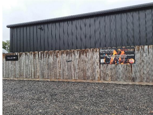
Figure 8 Proposed storage building already in situ
