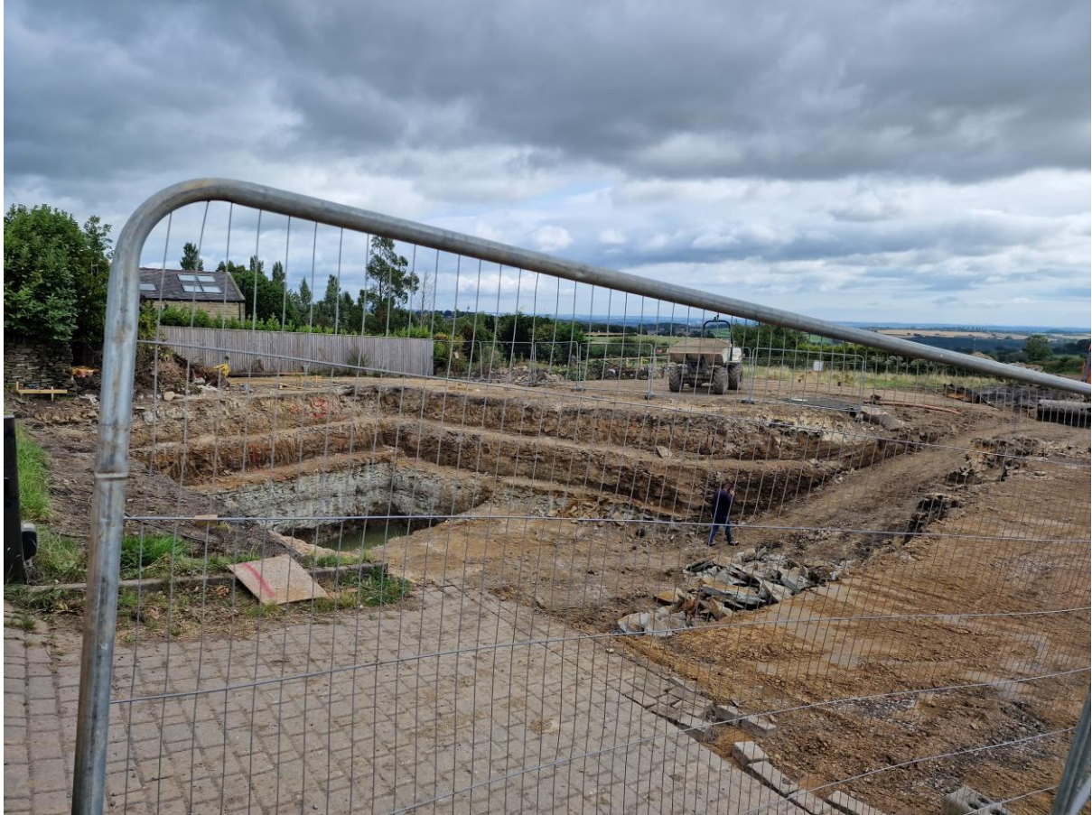
Photo 1: Site at time of excavation of basement – View from Sringer House lane
