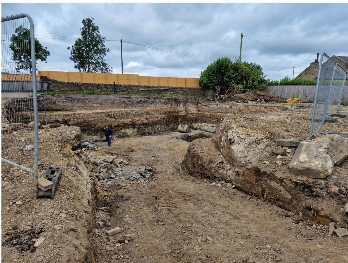
Photo 2: View towards Stringer House Lane – Excavation of Basement
