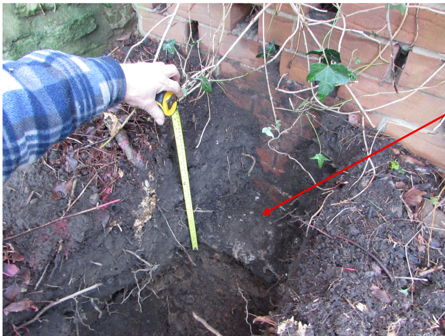
Photo 3 – Foundation of lighter wall structure, approximately 3.4 metres away from T5.
