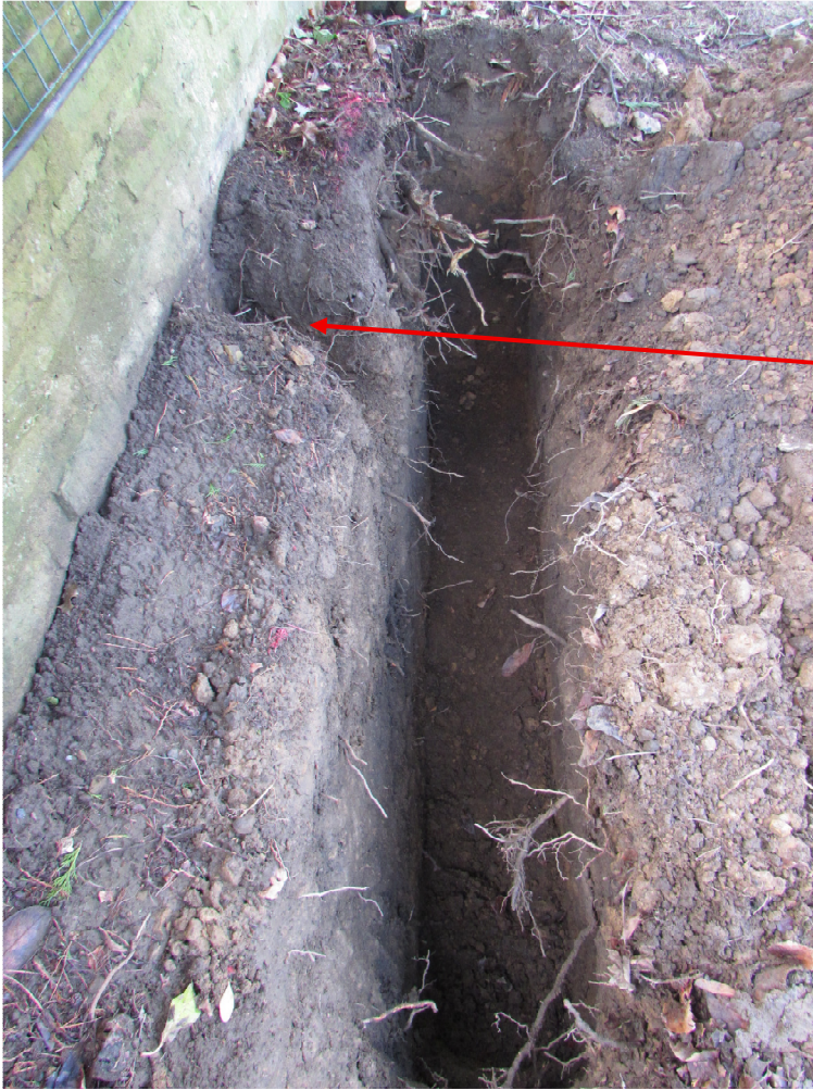
Photo 6 – Trial Pit 2 – Extent of roots in the trial pit
