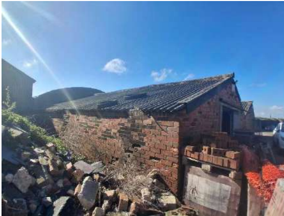
Photograph 3: Building B1 viewed from the north (22.04.2026).
