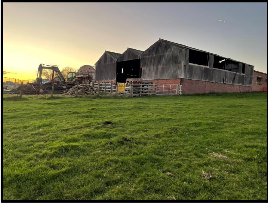
Photo 3 – Looking north west towards the site from the south east.
